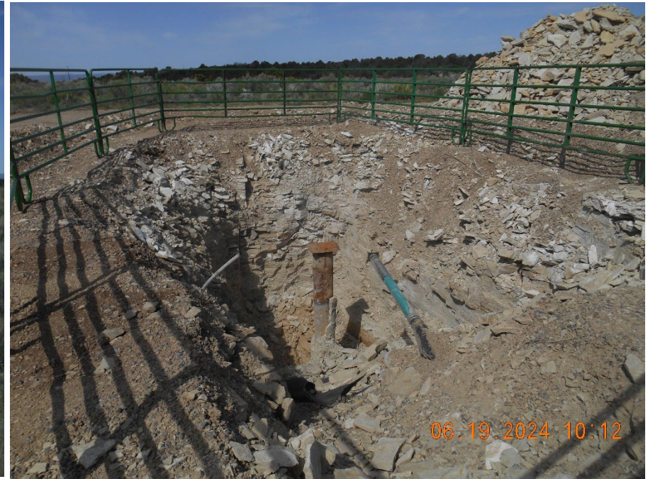
Injection Wellhead plugged and abandoned
