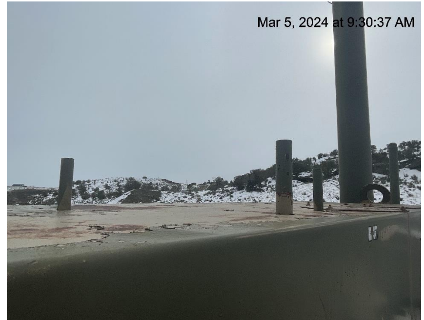
Photo # 8199 From inspection 708903205 conducted on 03/05/2024 PRV & rupture disc vent lines lack caps
