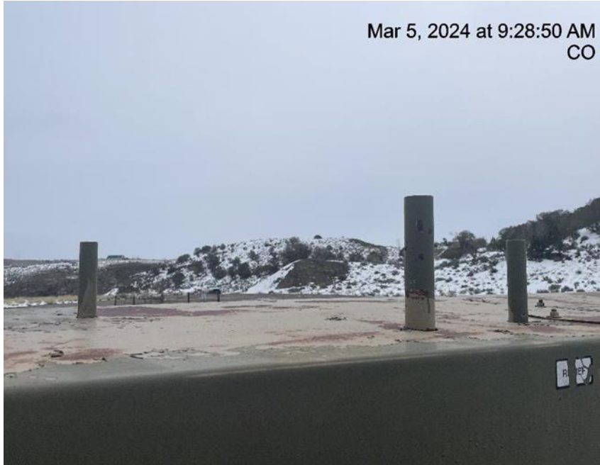
Photo # 8200 From inspection 708903205 conducted on 03/05/2024 PRV & rupture disc vent lines lack caps
