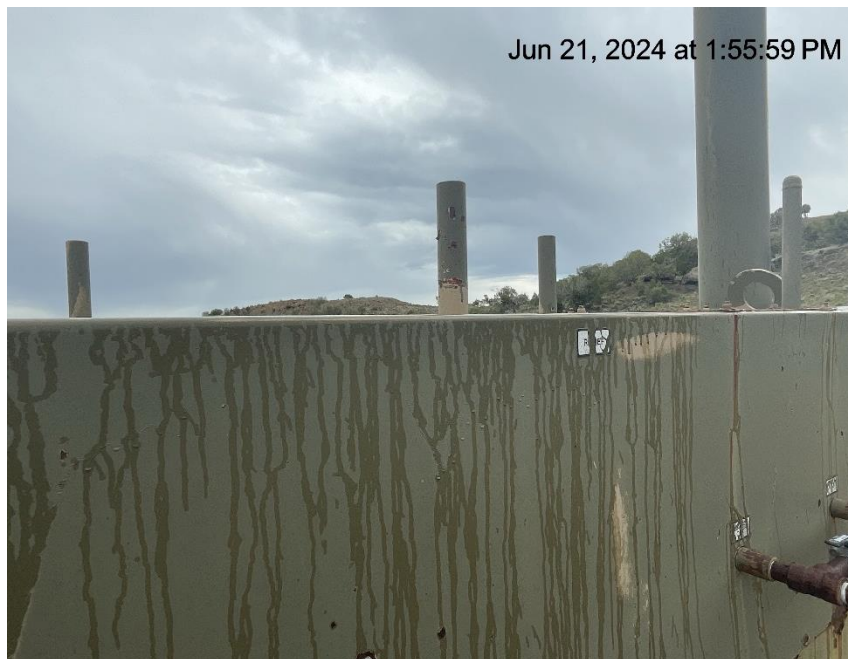
Photo # 1129 PRV & rupture disc vent lines lack caps
