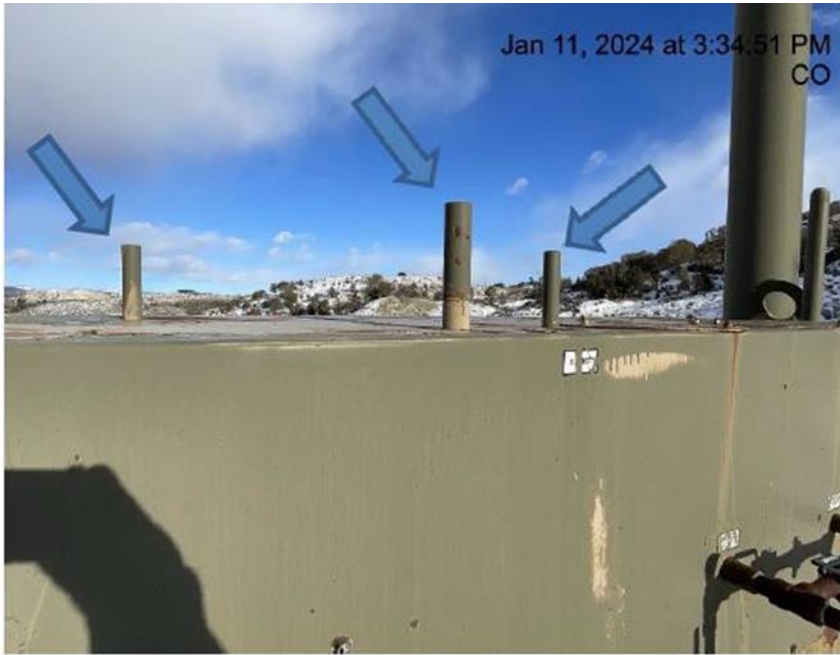
Photo # 2673 From inspection 708902787 conducted on 01/11/2024 PRV & rupture disc vent lines lack caps
