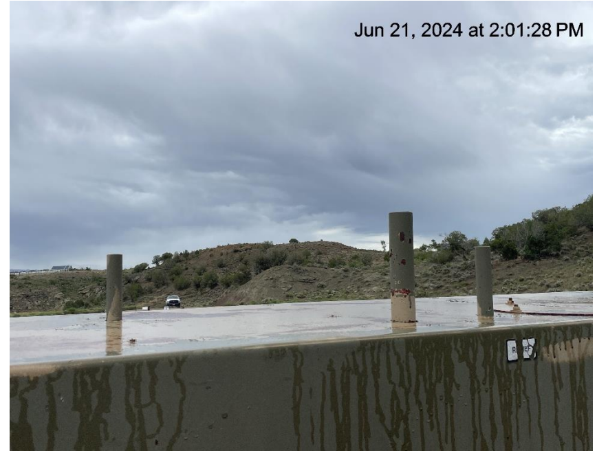
Photo # 1130 PRV & rupture disc vent lines lack caps
