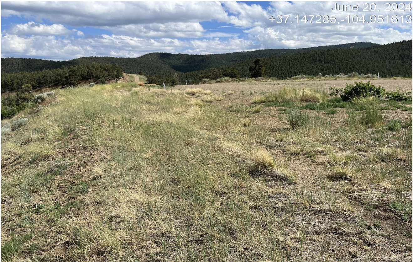
Photo 3. Facing south along the fill slope which is stabilized with vegetation.
