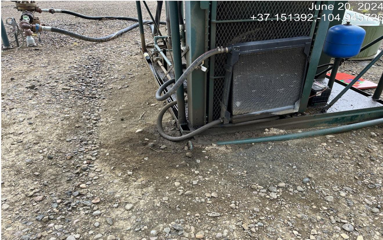
**Photo 3.** There is still oily fluid in the engine skid and stained soils.
