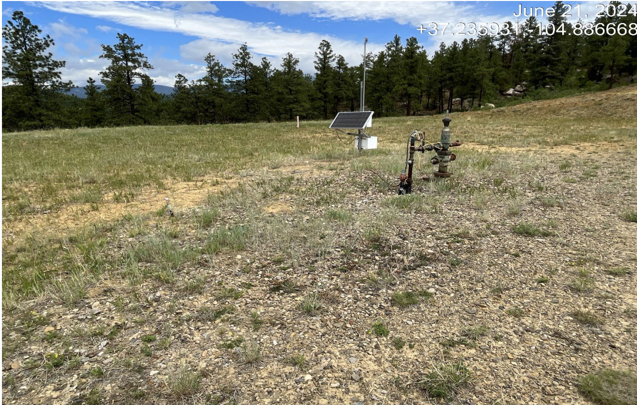
Photo 3. Facing toward the well which is temporarily abandoned..
