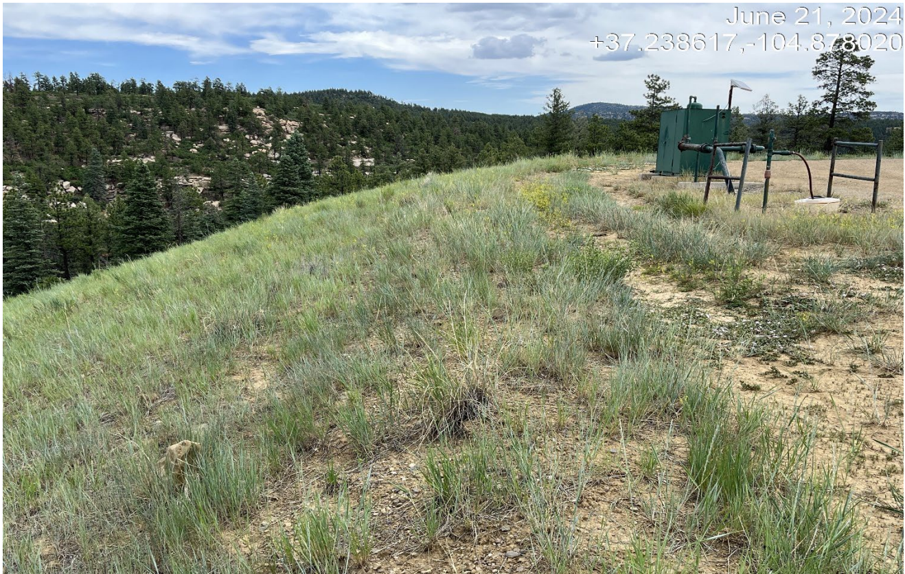
Photo 2. Facing east along the fill slope that is stabilized with perennial vegetation.
