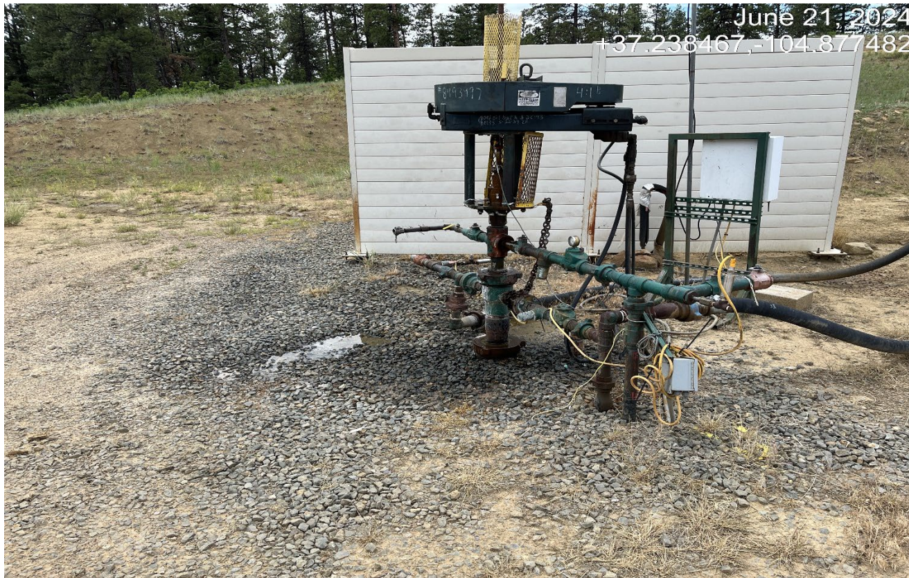
Photo 5. There is a dripping leak at the wellhead that needs to be fixed.
