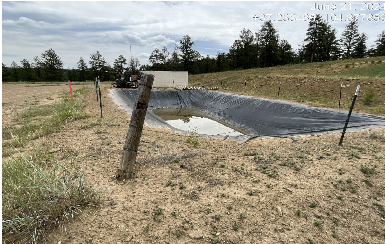
Photo 3. Facing toward production pit. The fence needs maintenance around the pit.
