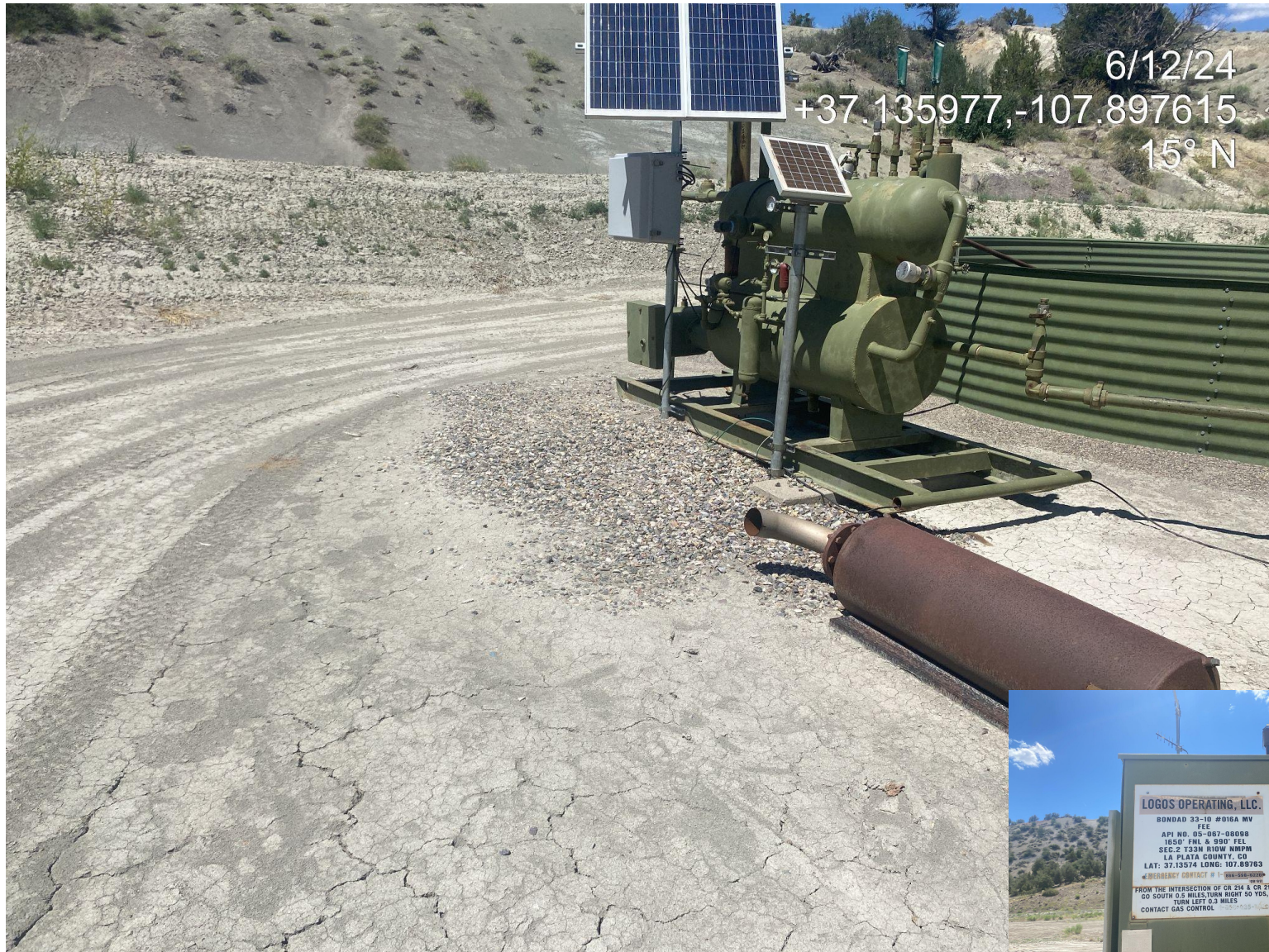
Photo 1. View of bondad 33-10 16A location on shared Simcoe location pad. Unused oil and gas equipment CA identified in the previous inspection doc #714000497 has been addressed/resolved.
