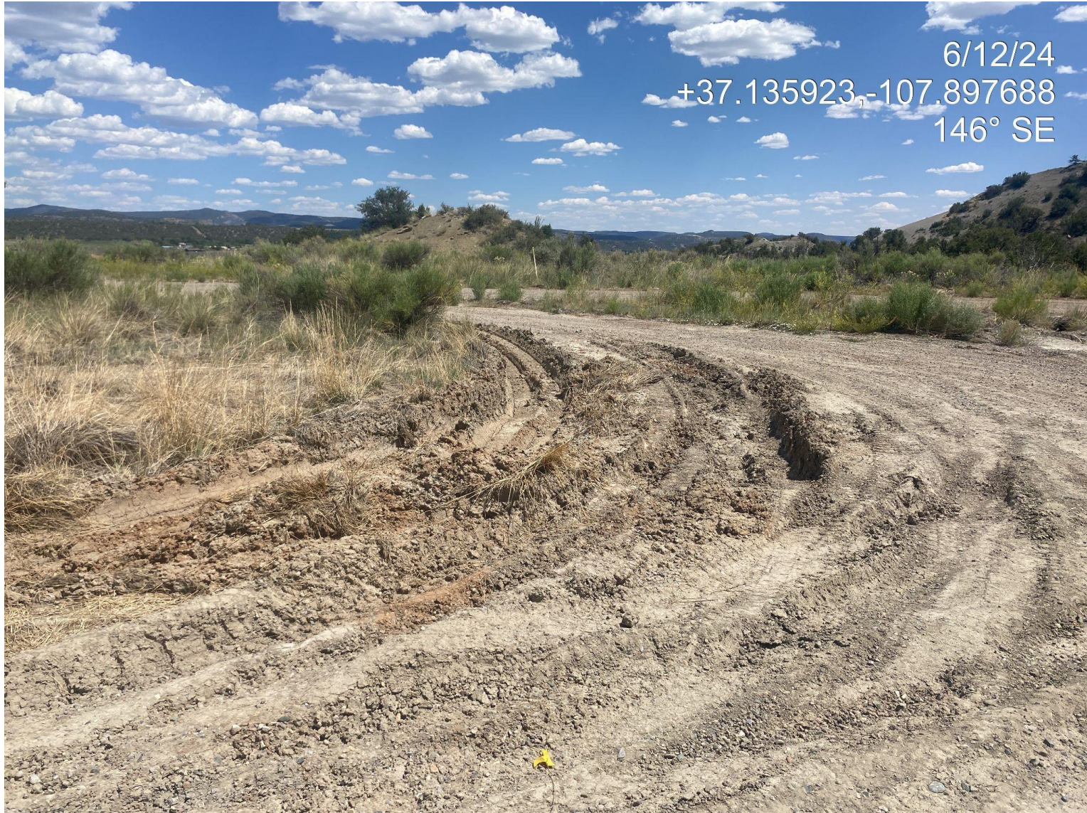
Photo 3. Deep rutting observed on the active pad near the Bondad 33-10 16A well. Additional stabilization/grading is needed to minimize degradation to the active pad.
