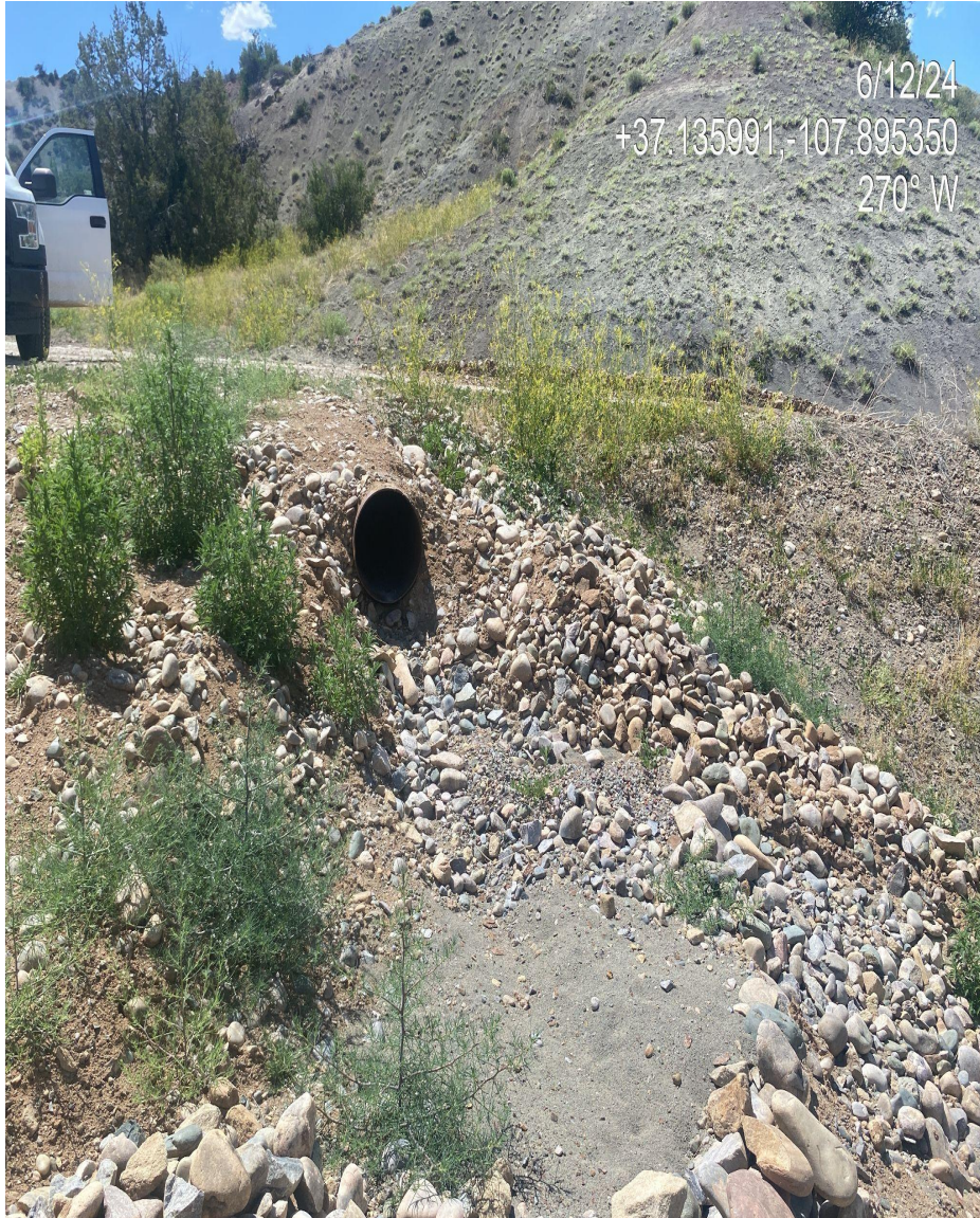
Photo 2. Storm water corrective action identified in the previous inspection doc #714000497 has been addressed/resolved.
