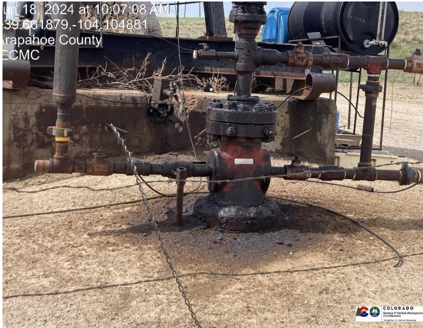
Pic 5 Stained soil around wellhead / mechanical issue
