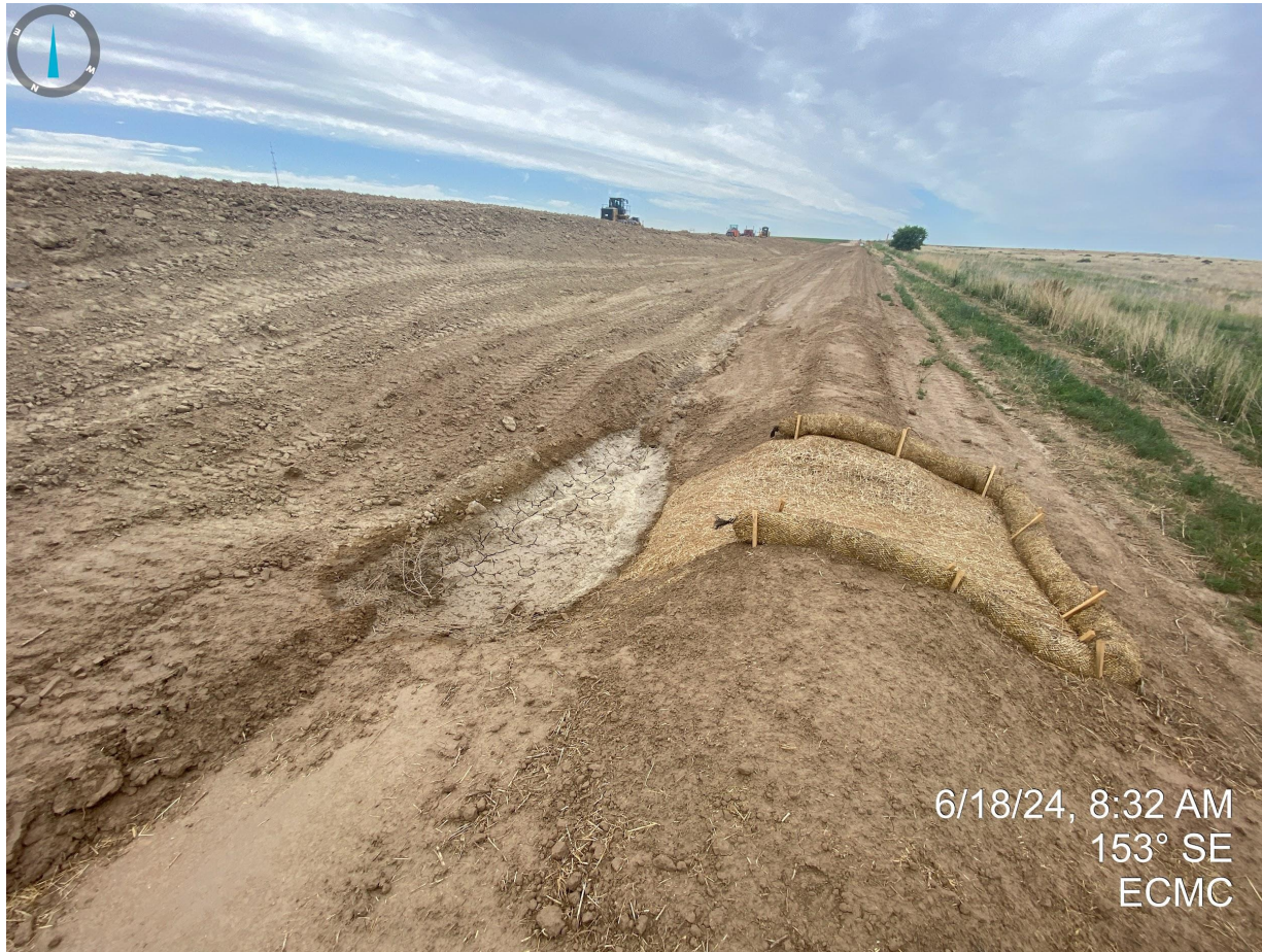
Photo 18. Ditch and berm with a sediment trap located on the west side of the location.
