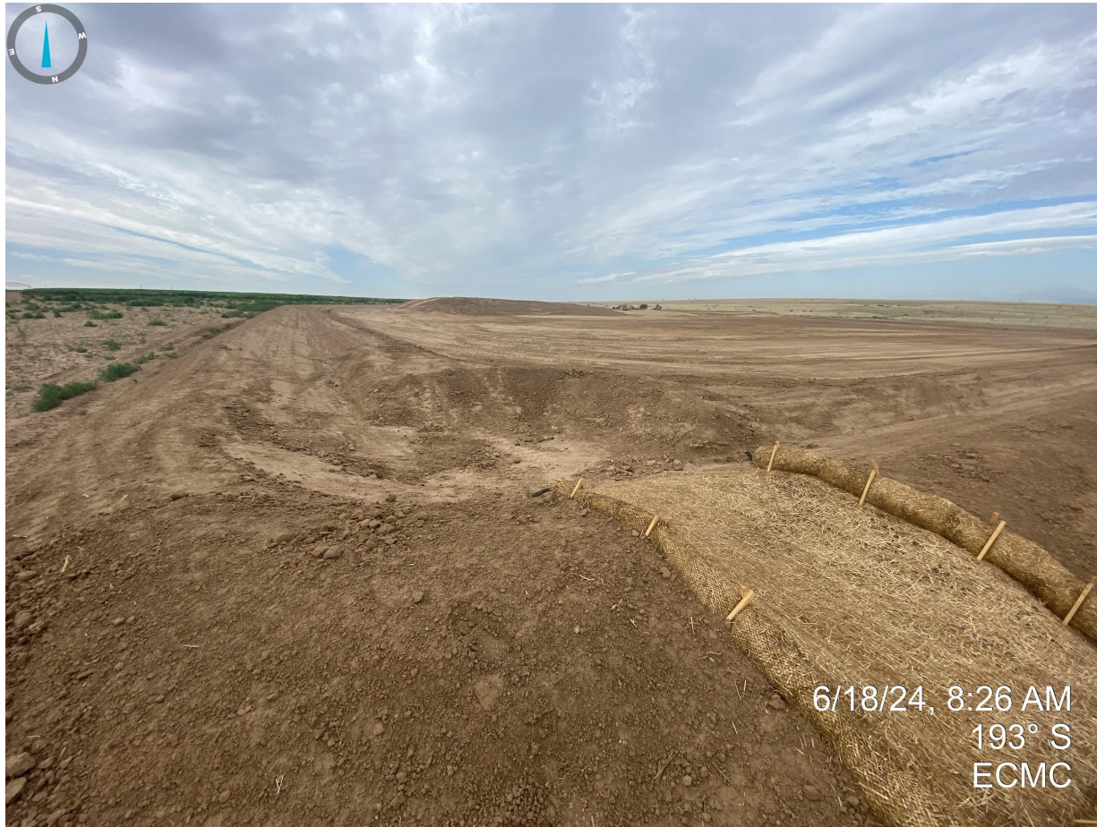
Photo 14. Northeast corner of the construction area; photo illustrates perimeter stormwater control measures (ditch and berm) have been installed around the entire location and sediment trap with temporarily stabilized outlet protection.
