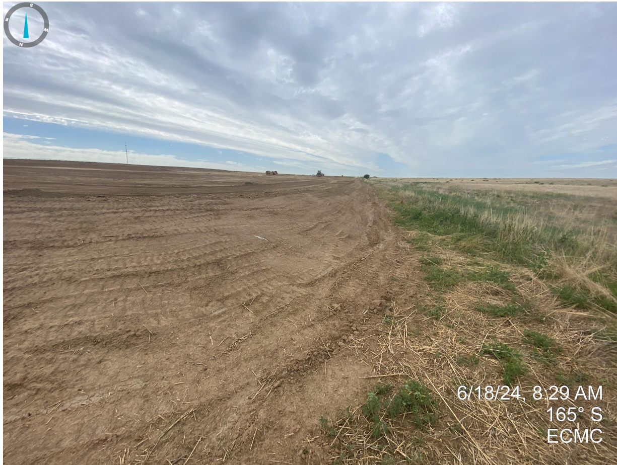
Photo 16. Northwest corner of the construction area; photo illustrates perimeter stormwater control measures (ditch and berm) have been installed around the entire location.
