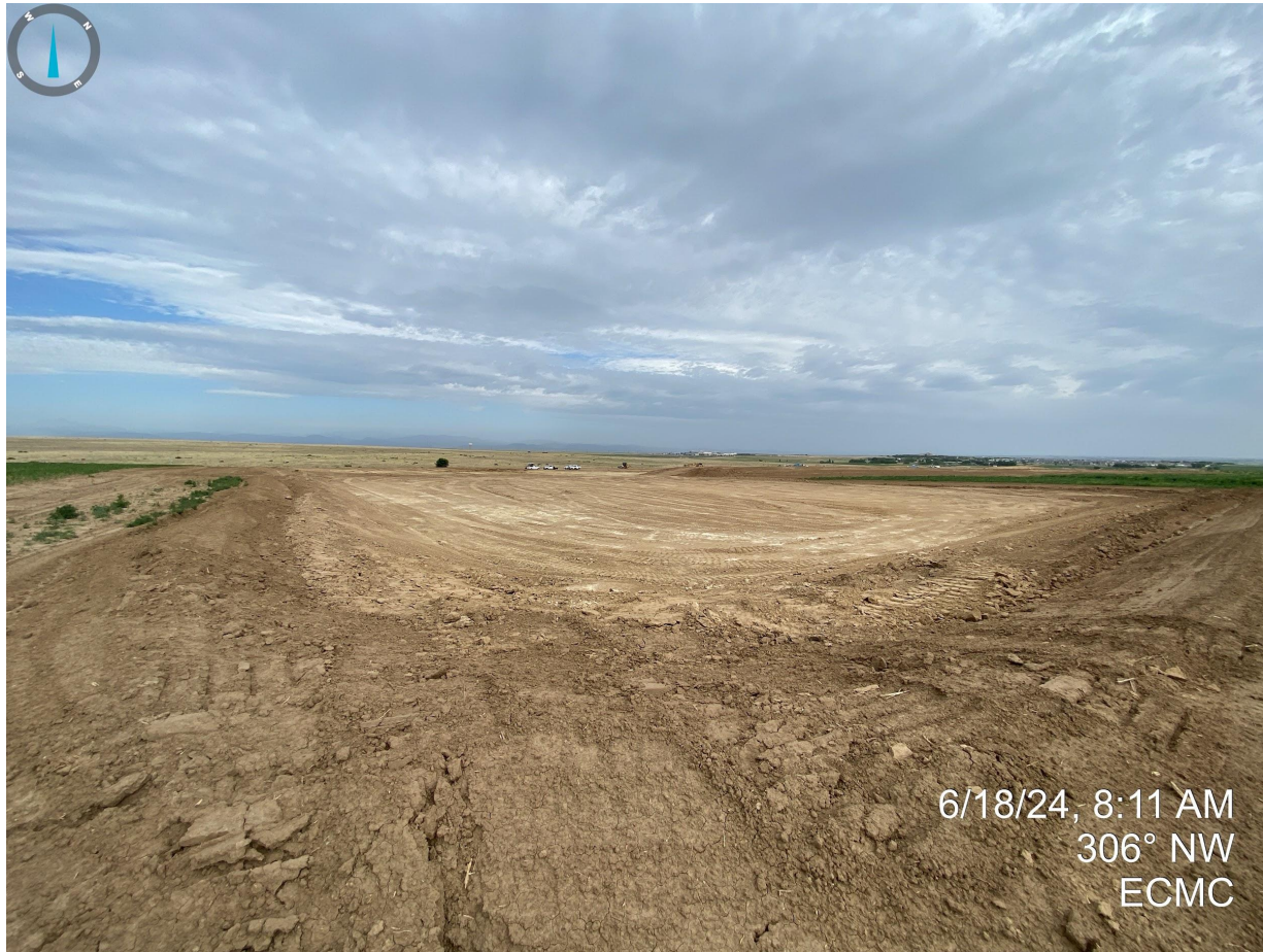
Photo 8. Taken from the southeast corner near the MLVT area. Perimeter stormwater control measures (ditch and berm) have been installed.
