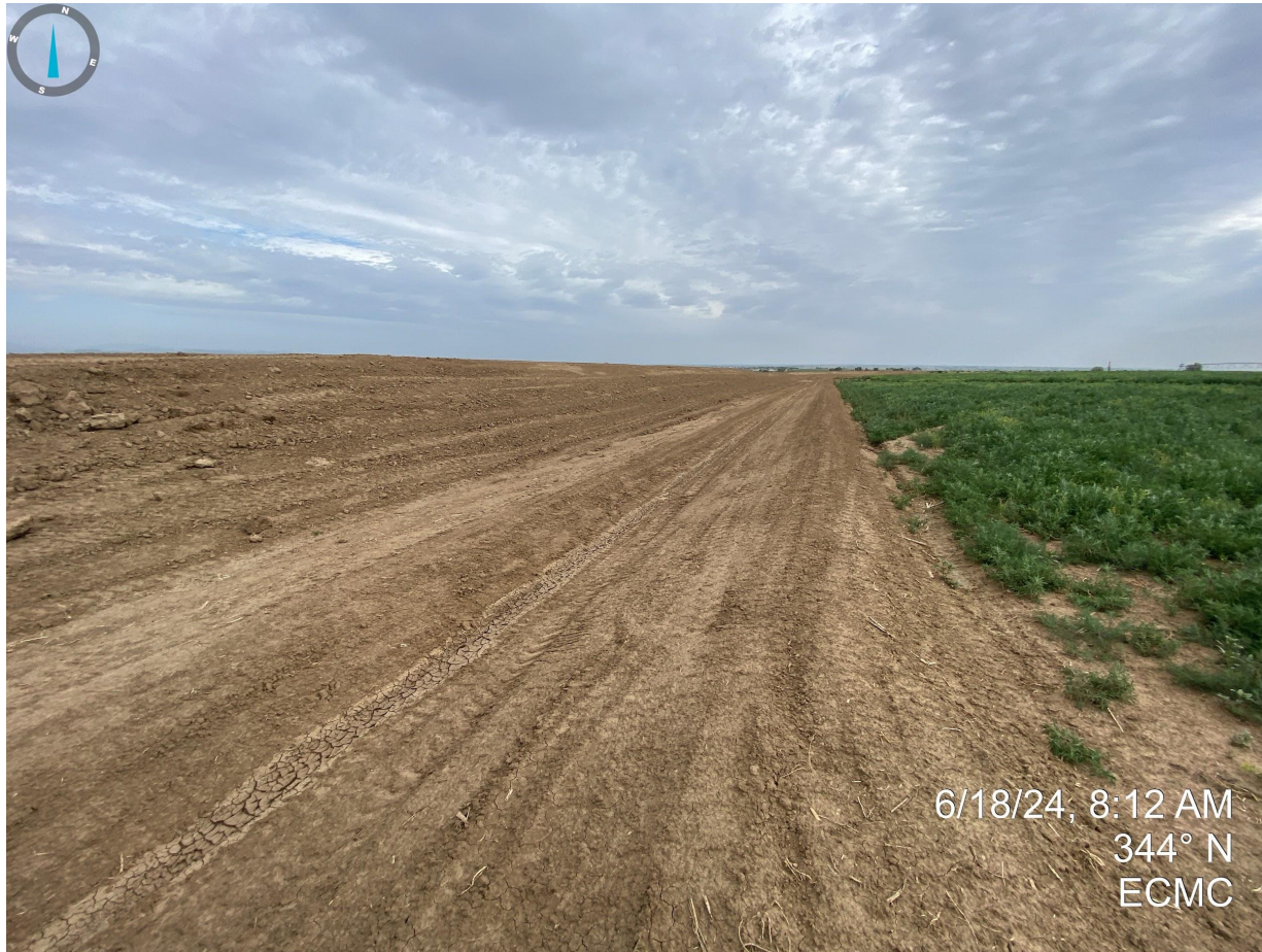
Photo 9. Taken from the east side of the construction area, facing north. Photo illustrates perimeter stormwater control measures (ditch and berm) and the topsoil stockpile area.
