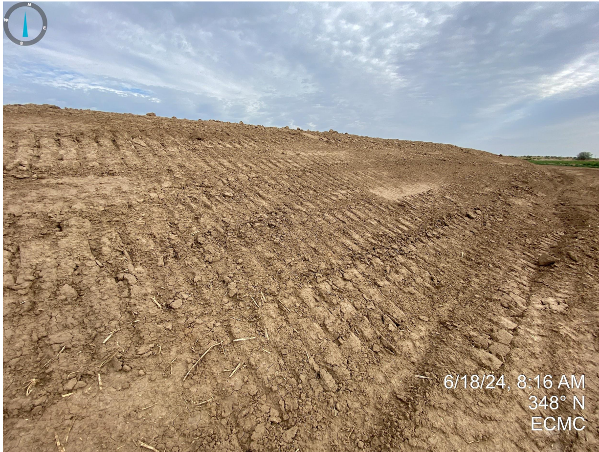
Photo 11. Eastside of construction area, facing north. Topsoil stockpile has been temporarily stabilized with equipment tracking, however, it has been installed parallel to grade. Long term stabilization techniques should be implemented (e.g. seeding).
