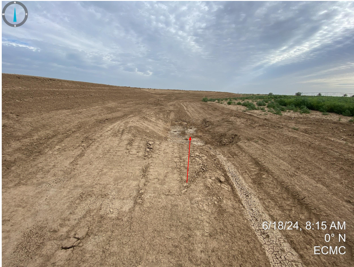
Photo 10. East side of construction area, facing north. Photo illustrates sediment trap that appears to be under construction.
