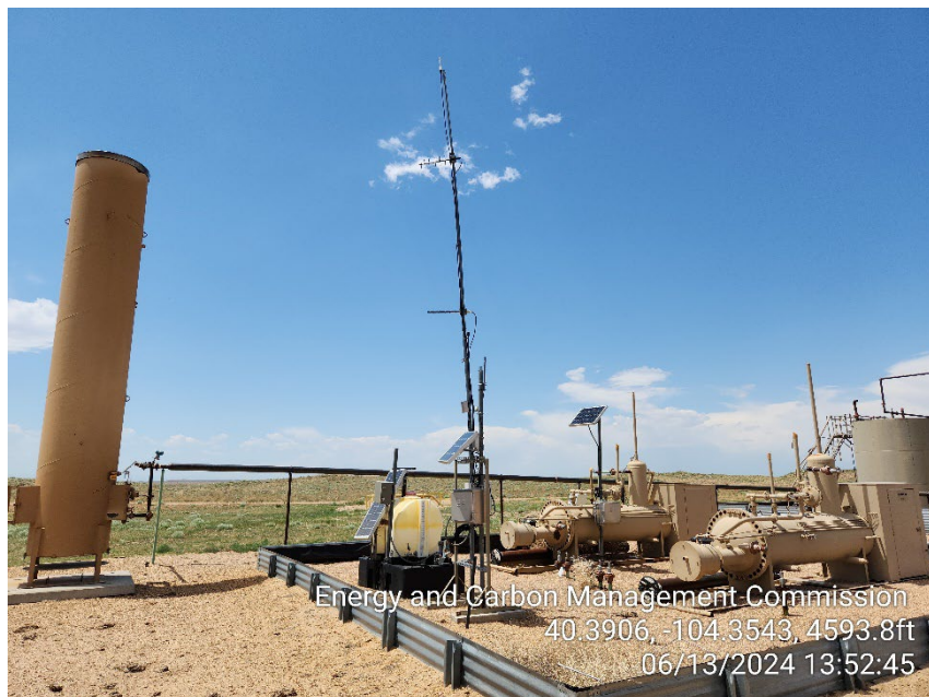
Photo 5 – Separators and ECD – Risers
