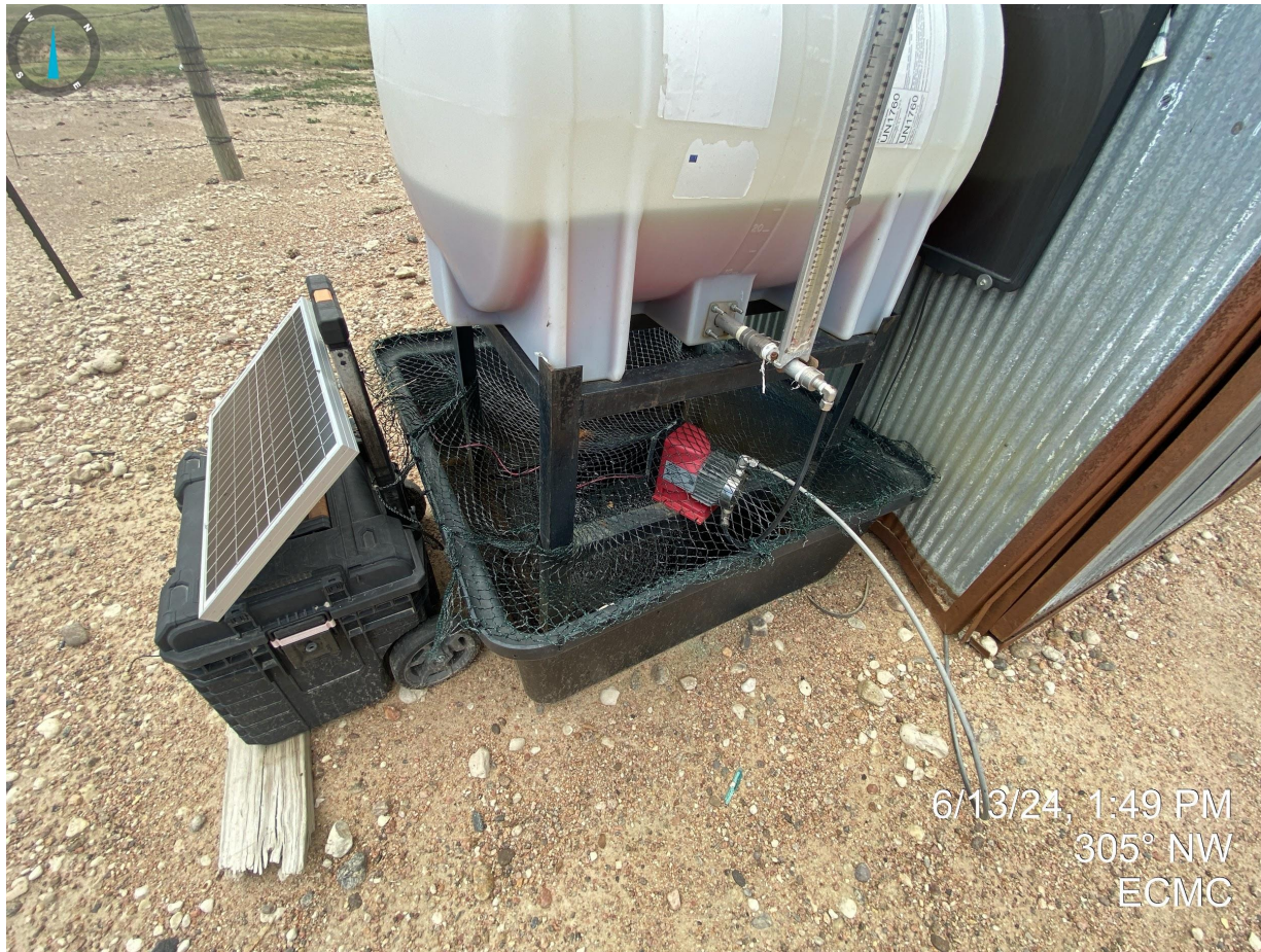
Photo 12. Free fluids observed within secondary containment have not been properly disposed of.
