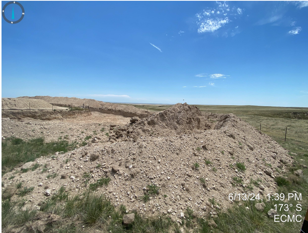
Photo 13. Taken from the north side of the stockpiled soils. No perimeter stormwater control measures/BMPs, or impermeable liners underneath the stockpile were observed during this inspection. Impacted soils appear to have been placed directly on top of undisturbed lands. Additionally, it does not appear that topsoil has been salvaged Per Rule 1002.b prior to stockpiling the soil on undisturbed portions of land.
