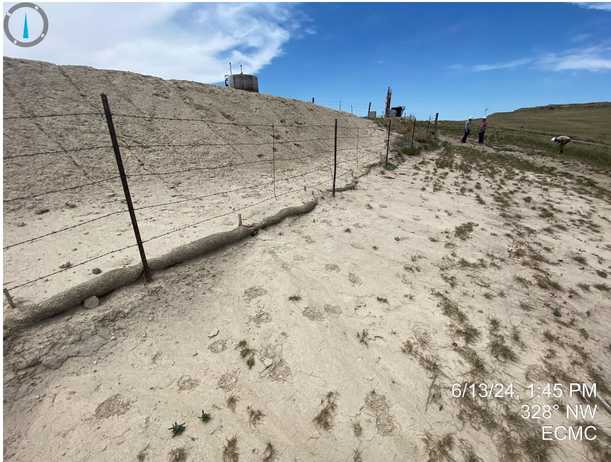
Photo 21. East side of pit; Stormwater control measures around the pit remain inadequate.
