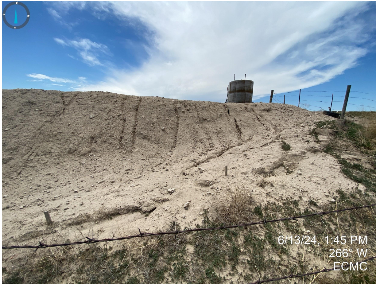
Photo 23. Northeast corner of the pit; erosion degradation pictured. Stormwater control measures around the pit remain inadequate.
