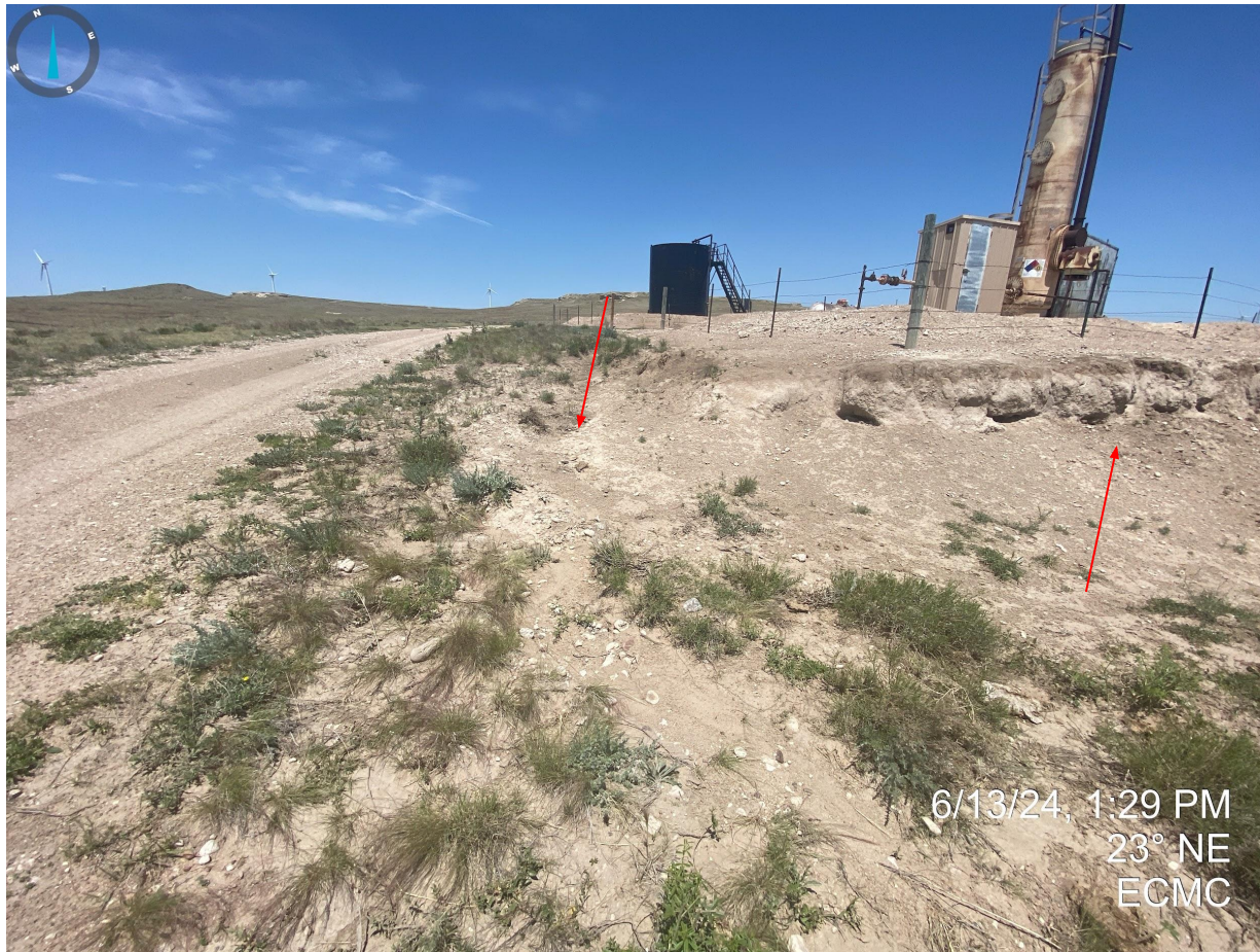
Photo 1. Areas experiencing erosion degradation throughout the production areas do not appear to have been repaired/stabilized and there is no evidence of stormwater controls measures/BMPs having been implemented.
