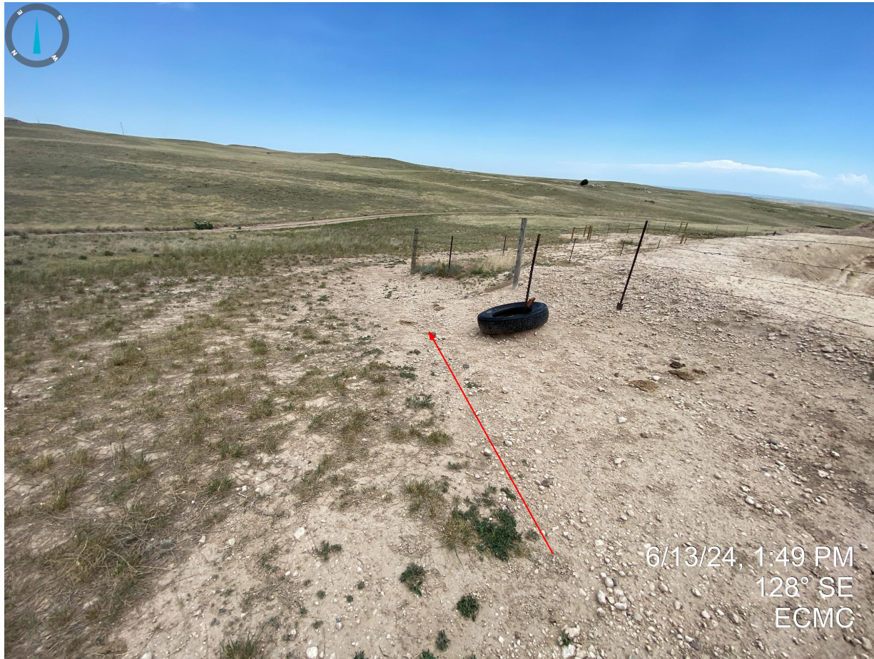
Photo 10. Erosion degradation occurring along the production areas; see comments in Photo 2.
