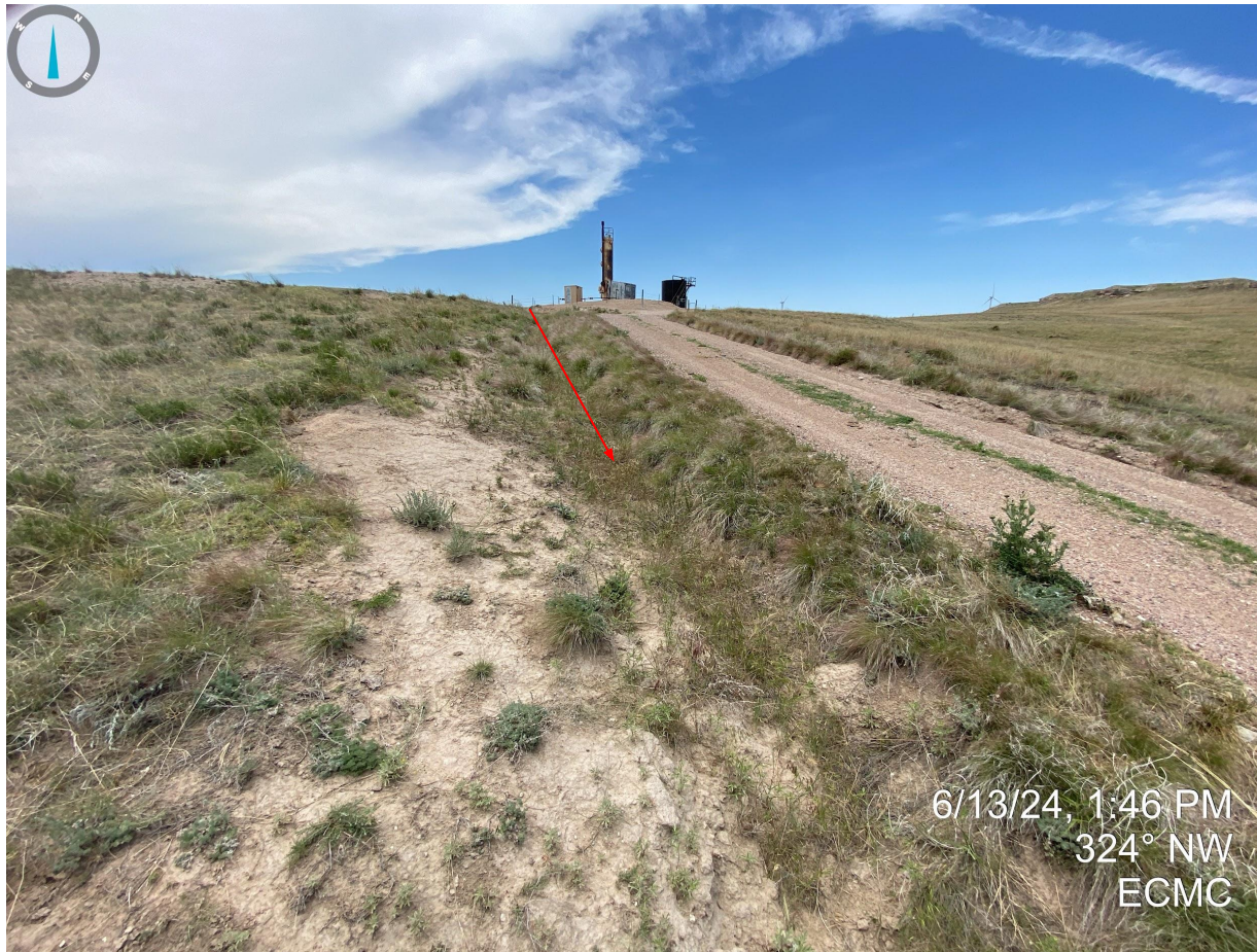
Photo 2. Taken from the access road east of the pit. Evidence of erosion degradation, previously documented, does not appear to have been repaired/stabilized with no evidence of control measures/BMPs observed that would prevent further erosion of the access road.
