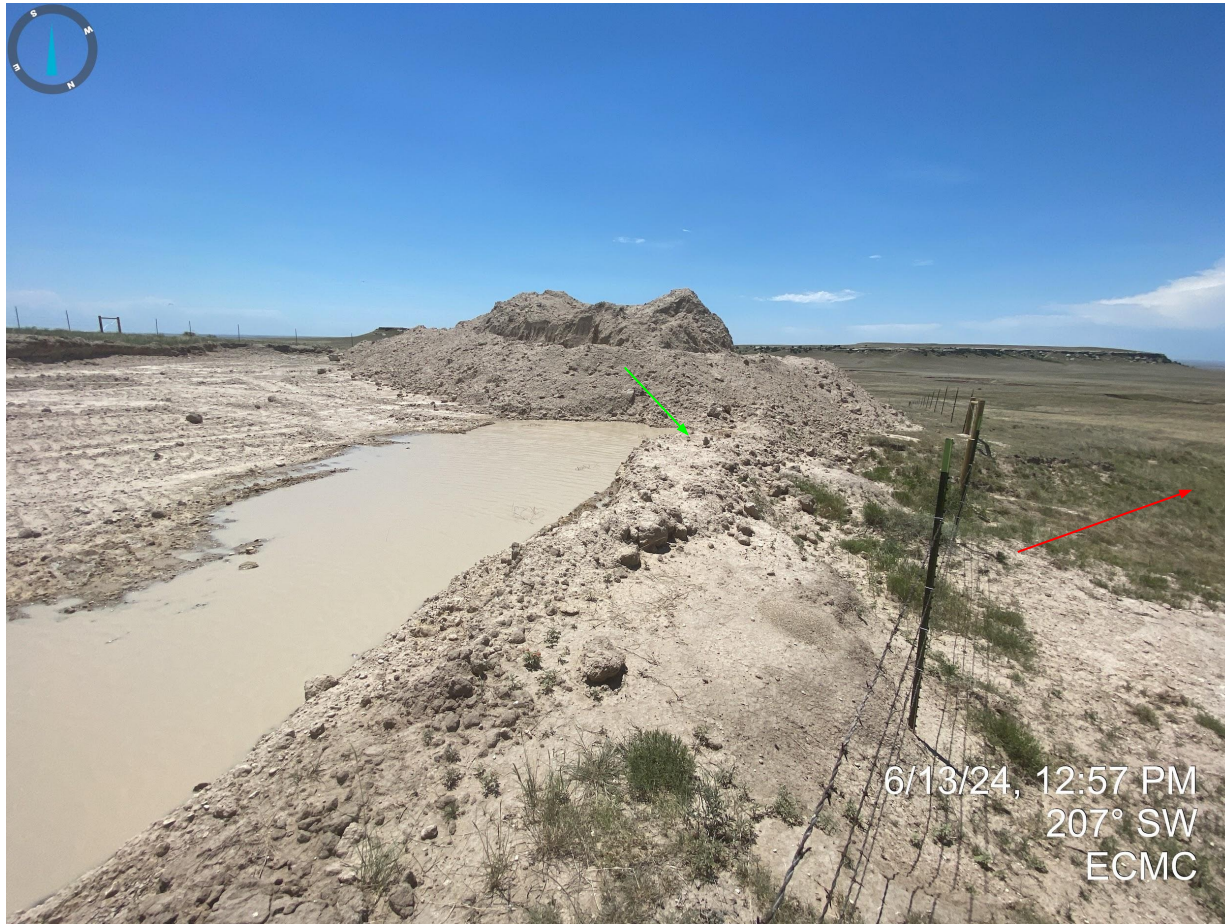
Photo 26. Continued from Photo 23. No stormwater control measures/BMPs were observed around the perimeter of the excavated area or stockpiles that would prevent off location stormwater discharge from entering nearby drainage (indicated by red arrow). Stormwater is close to spilling over the excavated area, indicated by green arrow.
