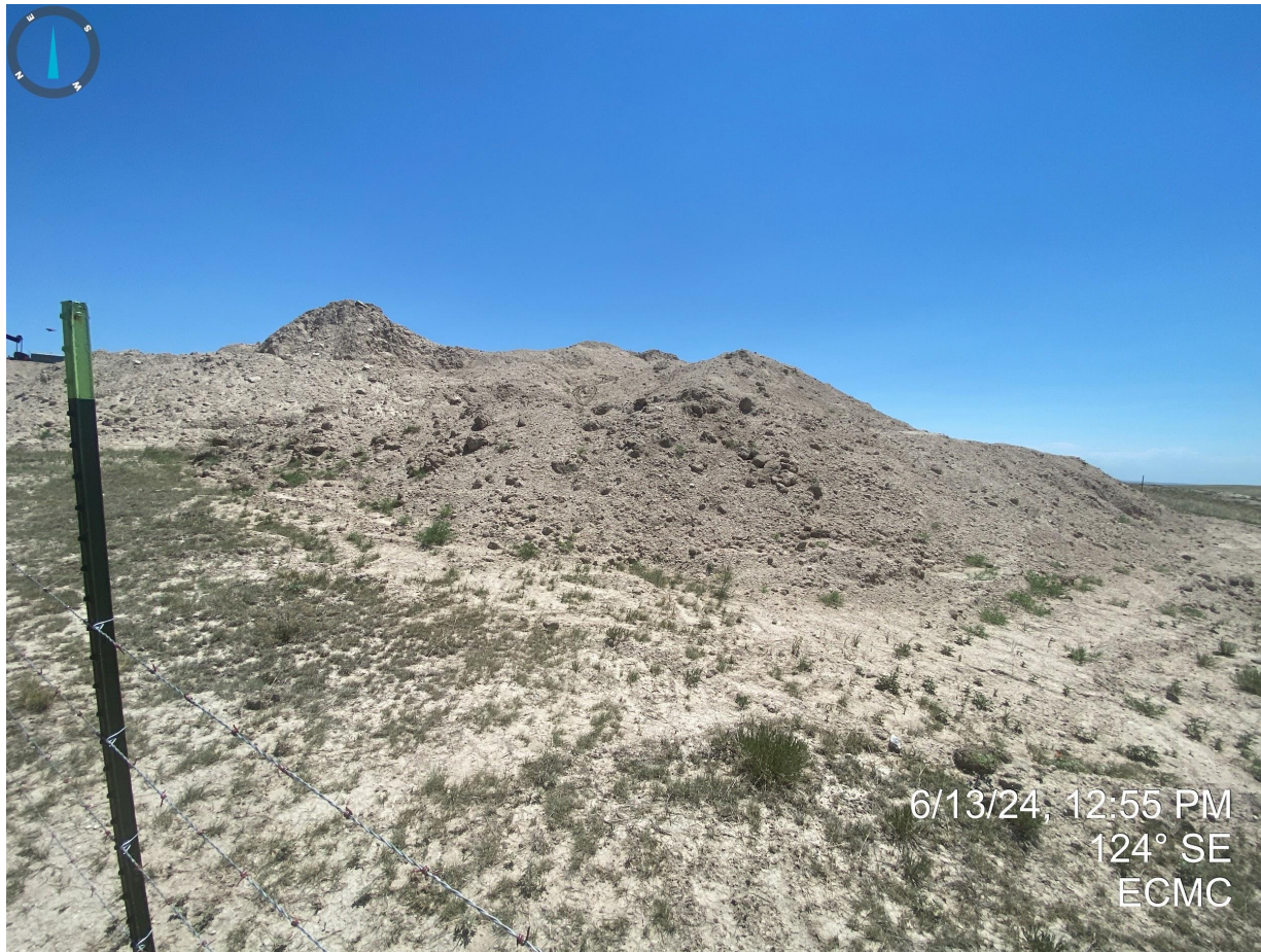
Photo 23. North side of excavation. No stormwater control measures/BMPs were observed around the perimeter of the excavated area or stockpiles that would prevent off location stormwater discharge from entering nearby drainage.
