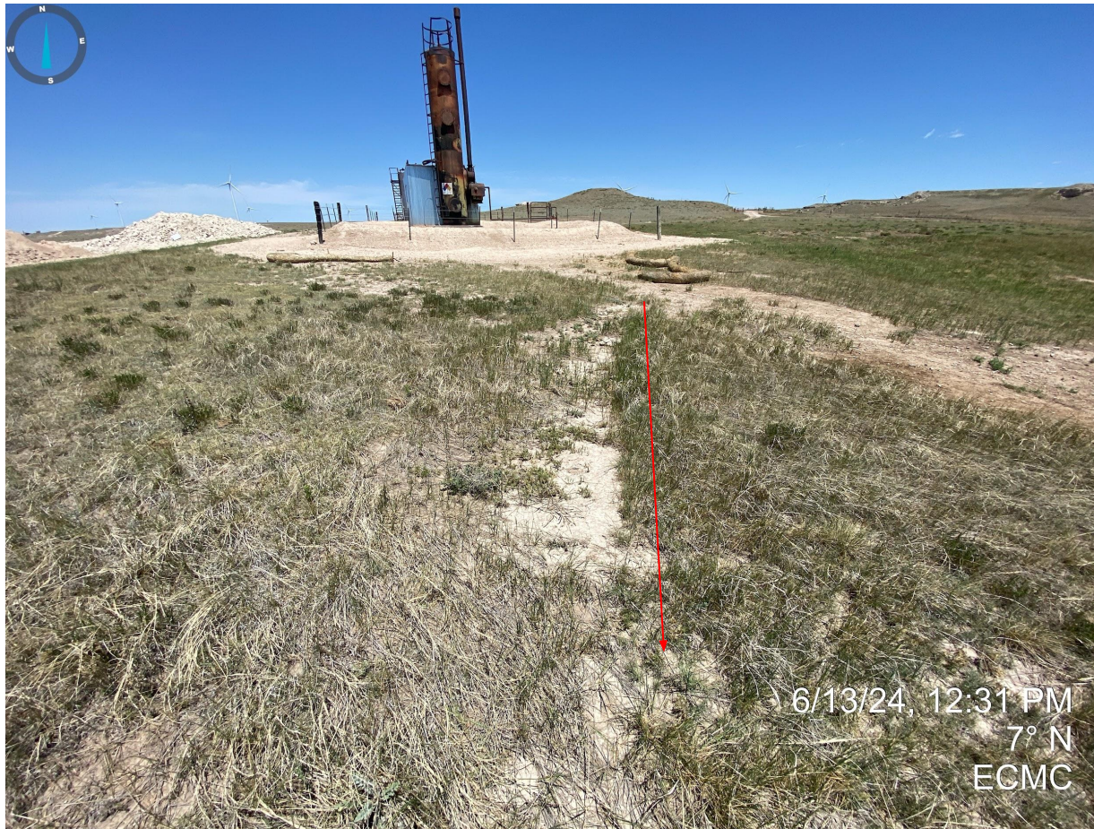
Photo 9. Sediment deposition observed south of the vertical heater treater. Stormwater control measures remain inadequate to prevent continued erosion degradation.
