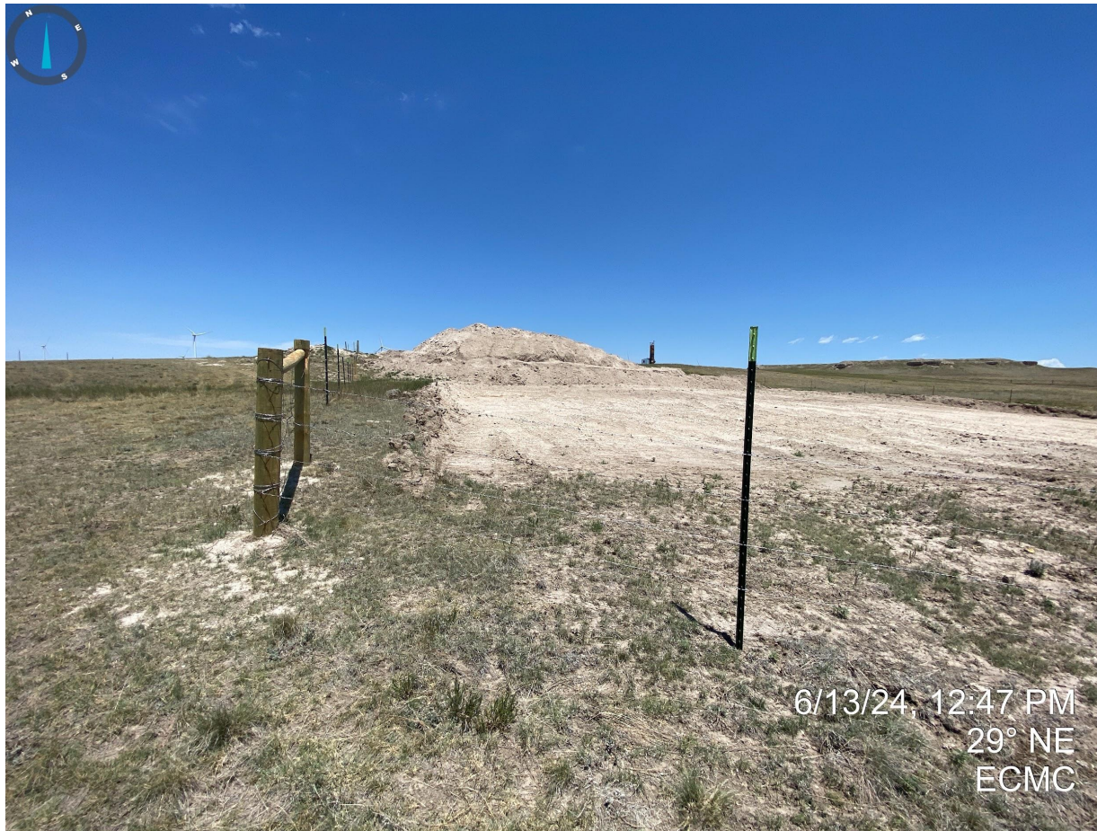
Photo 19. Fencing has been installed around the perimeter of the excavation and stockpiled soils. No perimeter stormwater controls/BMPS observed around the stockpiled soils or excavated areas.
