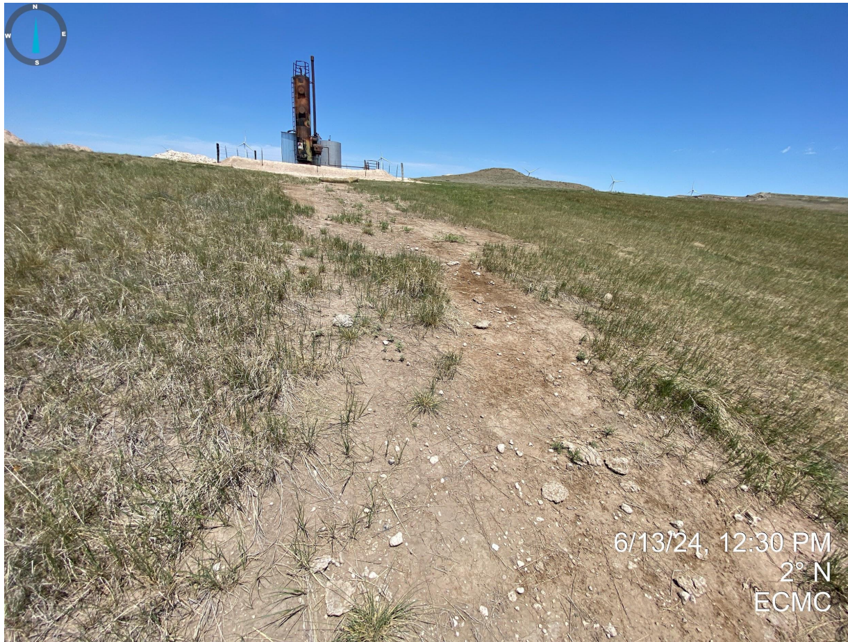
Photo 10. South of vertical heater treater. Photo illustrates unstabilized soils and lack of proper stormwater controls measures that would prevent erosion degradation.
