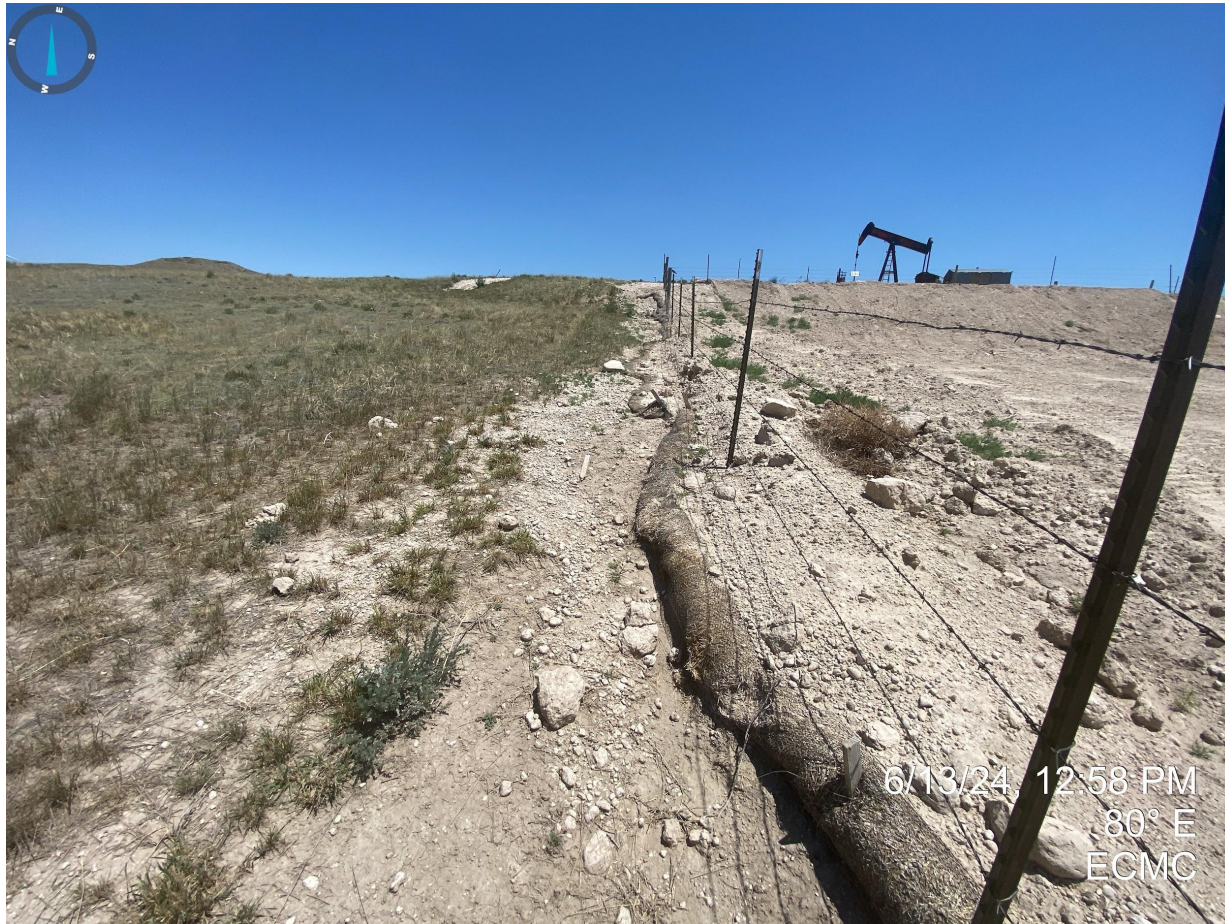
Photo 27. Taken from the north side of the pit. It does not appear that any erosion degradation has been properly stabilized or repaired, and stormwater control measures remain inadequate as the straw wattles are degraded and not properly functioning.
