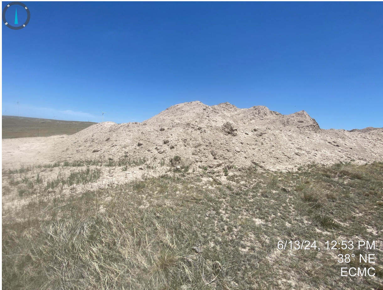
Photo 21. Western stockpiled material is not properly stabilized with evidence of unconsolidated materials. No perimeter stormwater control measures observed.
