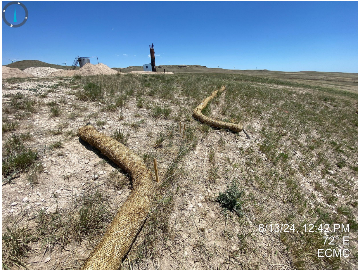
Photo 15. Straw wattles not properly installed.
