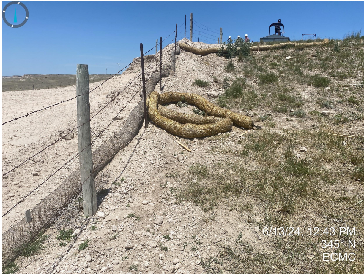
Photo 16. Erosion degradation doesn't appear to have been repaired and stabilized and straw wattles are not adequate.
