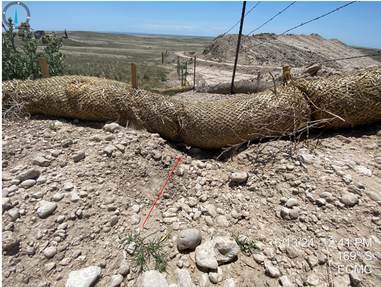
Photo 13. Close up of straw wattles not trenched and backfilled; daylight observed.
