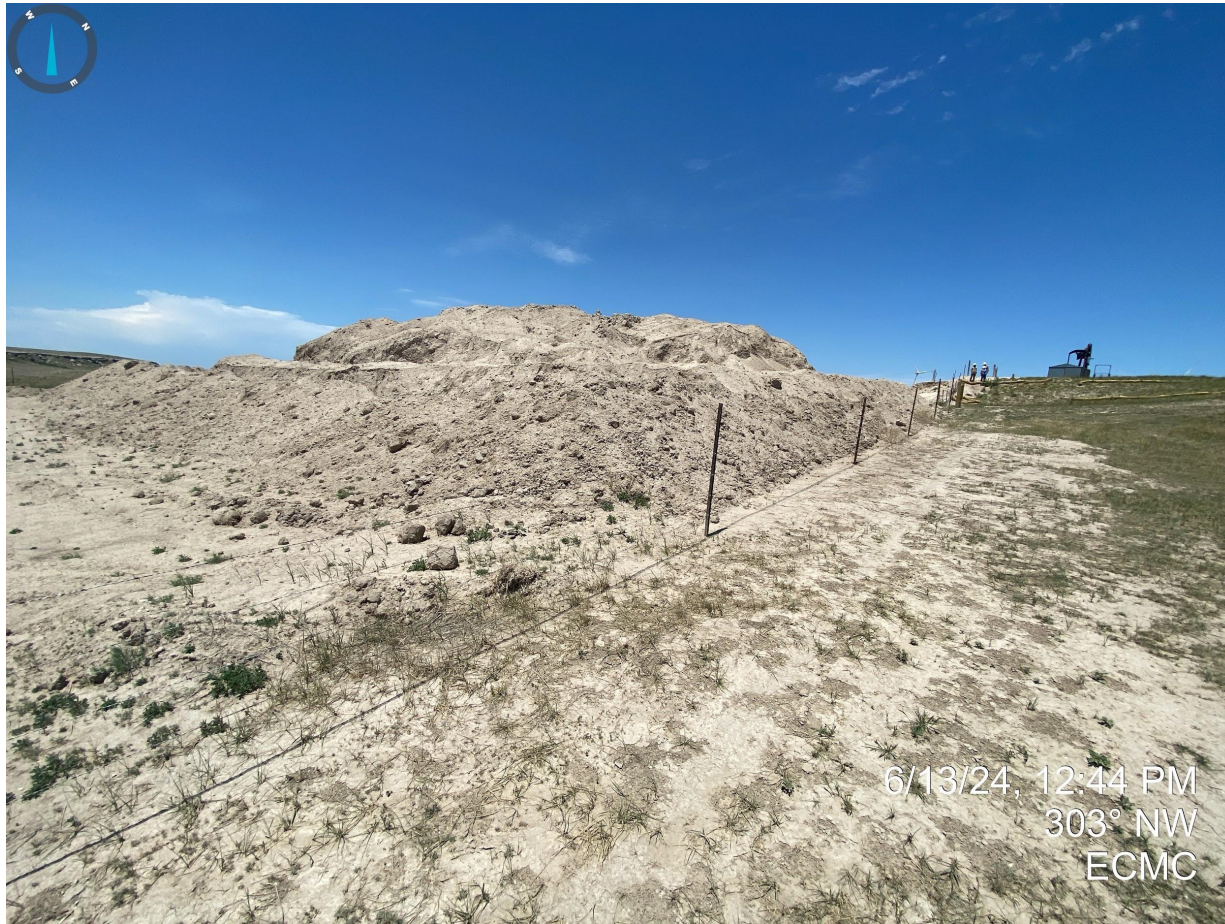
Photo 18. Fencing has been installed around the perimeter of the excavation and stockpiled soils. No perimeter stormwater controls/BMPS observed around the stockpiled soils or excavated areas.
