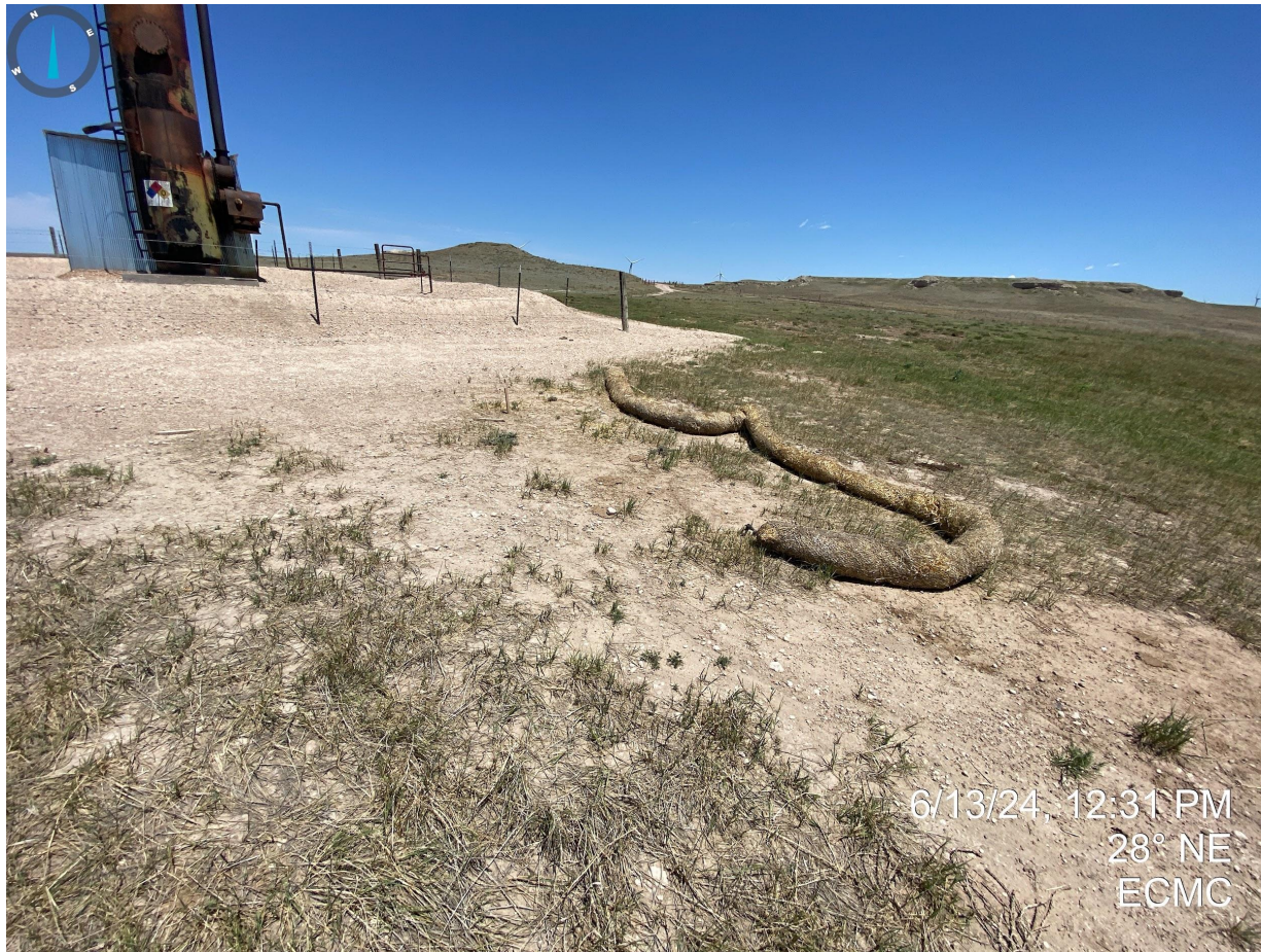
Photo 6. Facing northeast at the heater treater. Stormwater control measures (straw wattles) do not appear to be installed per good engineering practices (trenched and backfilled) and require maintenance.
