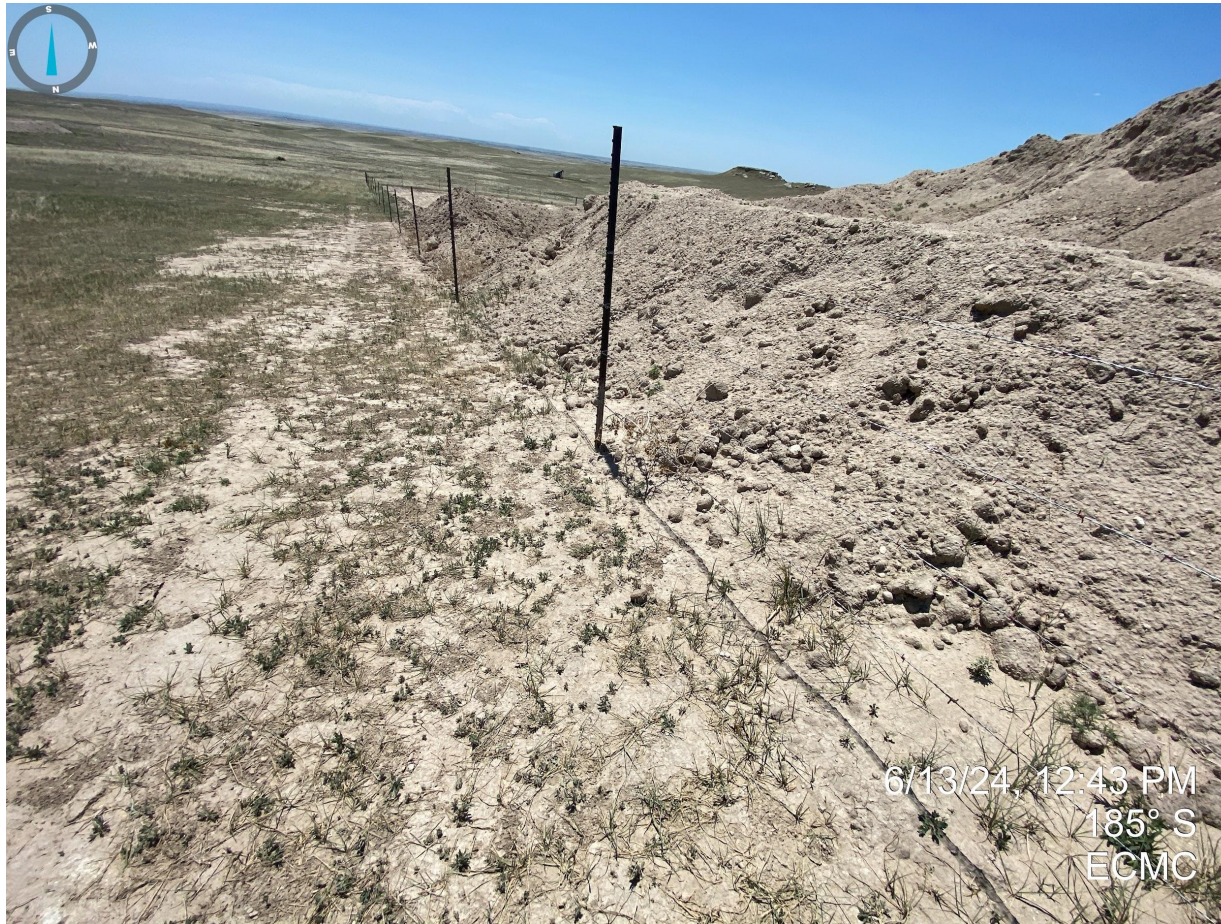
Photo 17. East side of stockpiled pit soils. Photo illustrates that both the stockpile and berms have been left unconsolidated. Unconsolidated materials can become a potential pollution source as it is not properly stabilized. Berms also appear to be built out of impacted material from the salt kill/pit excavation.
