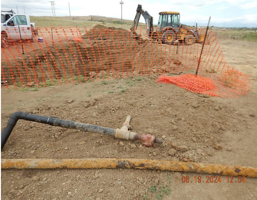
Flowline pipe and riser removed from excavation; mixed materials were observed that included CS, HDPE and fiberglass flowline pipe.
