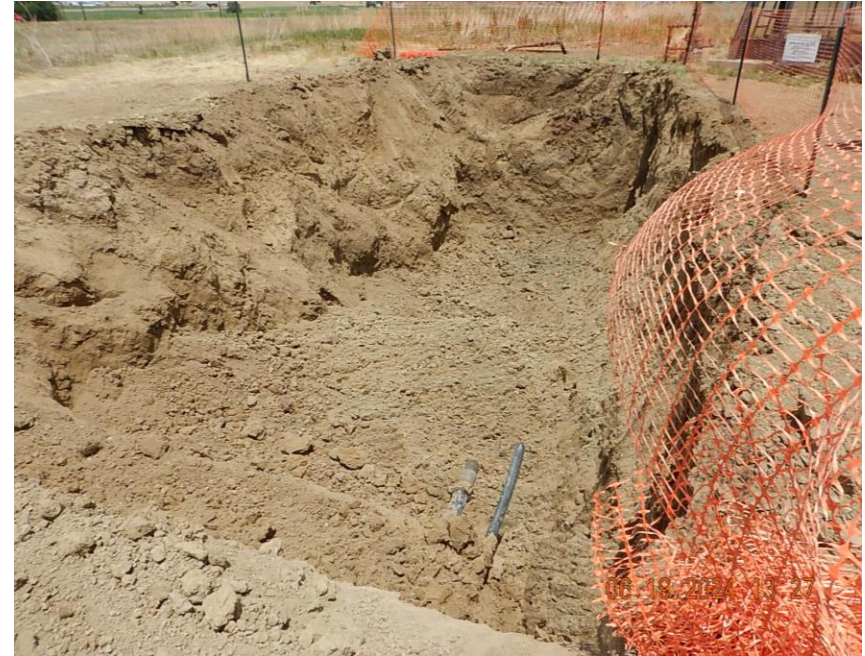
West side of fenced excavation looking east to wellhead. Flowlines exposed in excavation include (1) 3" fiberglass multiphase flowline (end bull plugged) and (1) 1.5" HDPE gas flowline.
