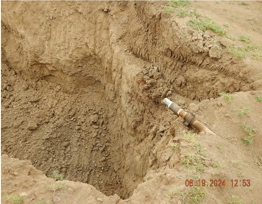
East side of excavation adjacent to wellhead. Flowline (2" CS OLF) cut end is bull plugged (end sealed).
