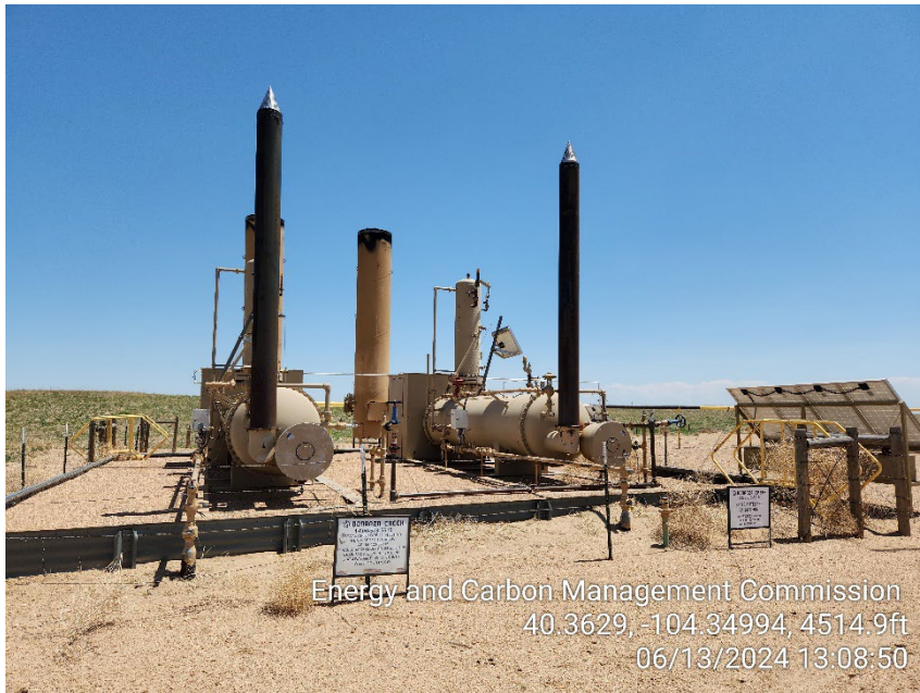
Photo 1 – Separators and ECDs
