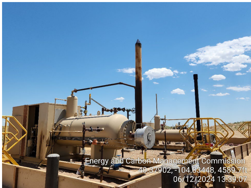
Photo 1 – Separators – Unmarked Risers in varies spots
