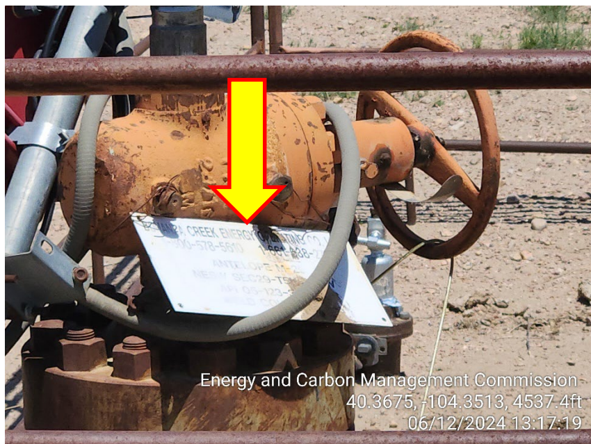
Photo 5 – Wellhead – Sign faded; no longer visible
