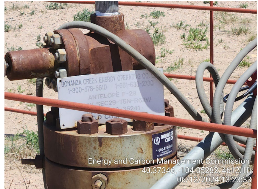
Photo 2 – Wellhead – Sign faded; no longer visible
