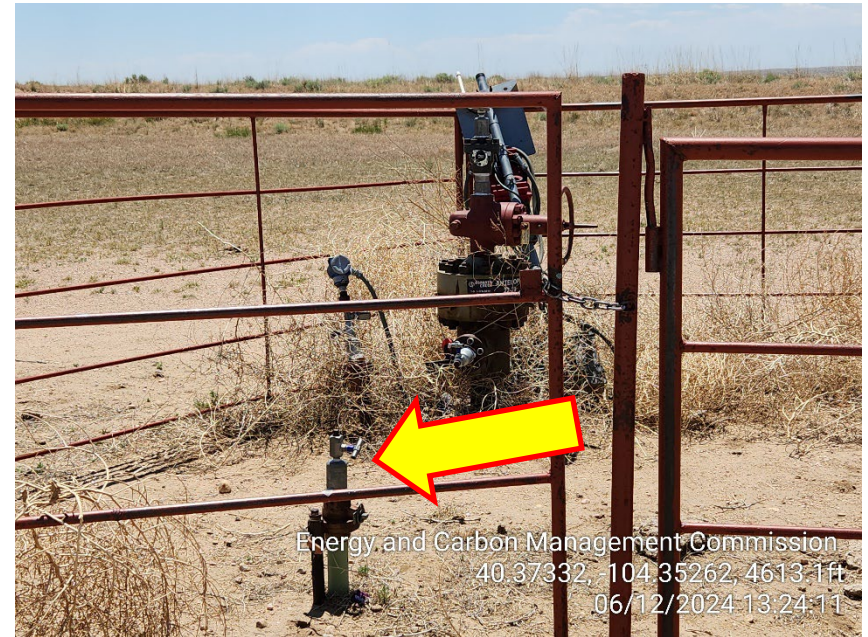
Photo 8 – Wellhead – Tumbleweeds and Unmarked Risers
