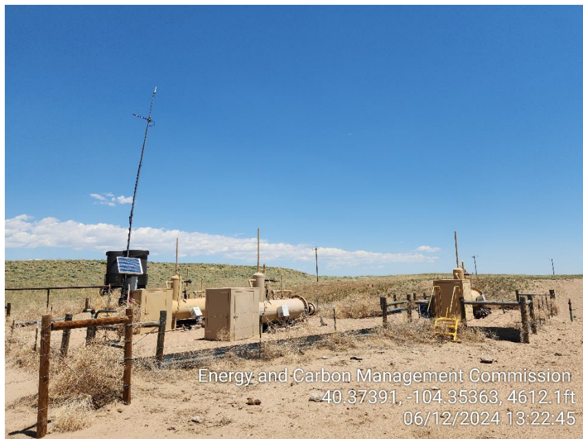
Photo 3 – Separators – Tumbleweeds
