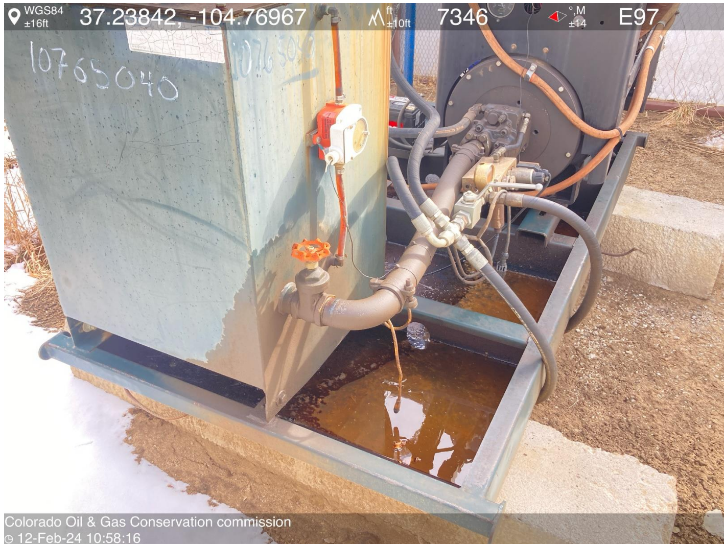
PHOTO 5: OILY WASTE IN ENGINE SKID. COMPLY WITH RULE 1002.f.(2)B, Comply with general provisions of the oil and gas act for wildlife protection AND SB-181. CA DATE 2-13-2024.
