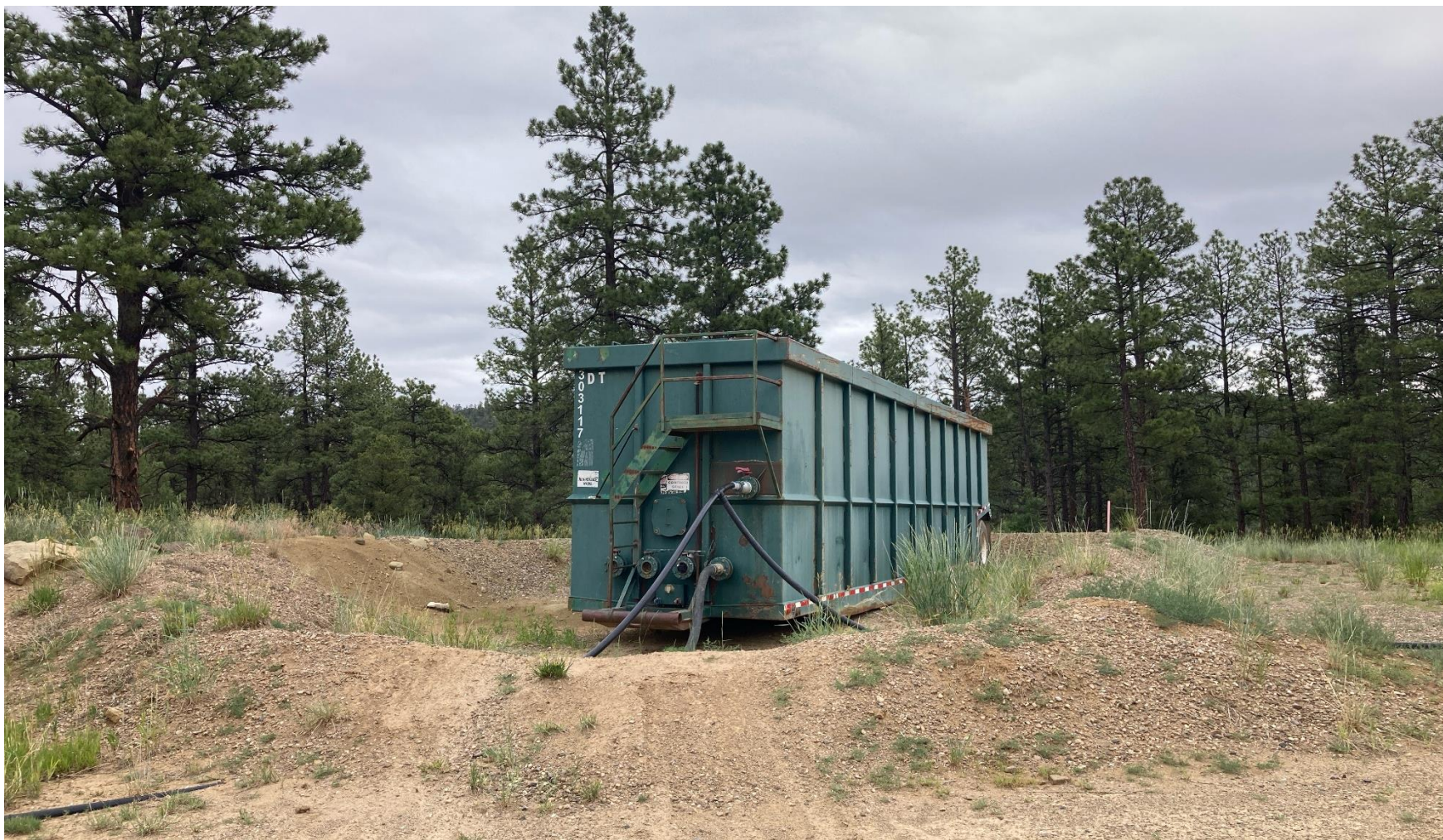
PHOTO 5: NO CAPACITY OR NFPA STICKER POSTED @ TANK BATTERY. Install sign to comply with Rule 605.h. CA DATE 7/19/2024.
