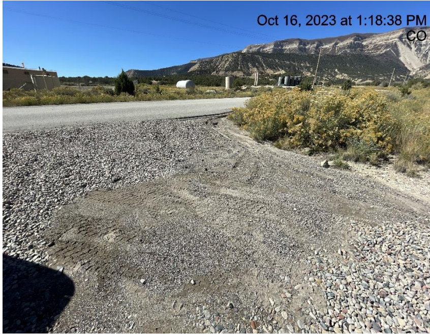
Photo # 2889 From inspection 708901973 conducted on 10/16/2023 Sediment migrating onto gravel track pad/BMP needs maintenance
