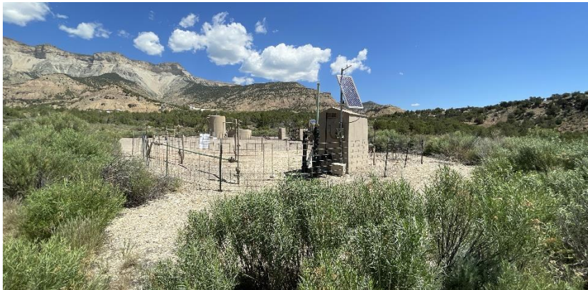
South West corner of location.
