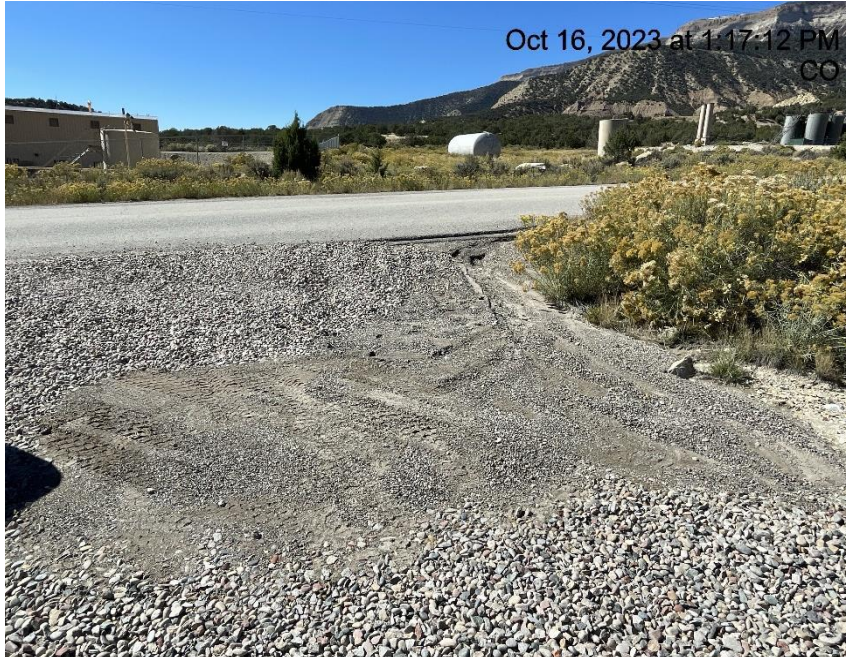
Photo # 2892 From inspection 708901973 conducted on 10/16/2023 Sediment migrating onto gravel track pad/BMP needs maintenance
