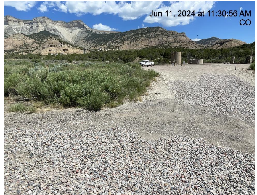
Photo # 438 Sediment migrating onto gravel track pad/BMP needs maintenance
