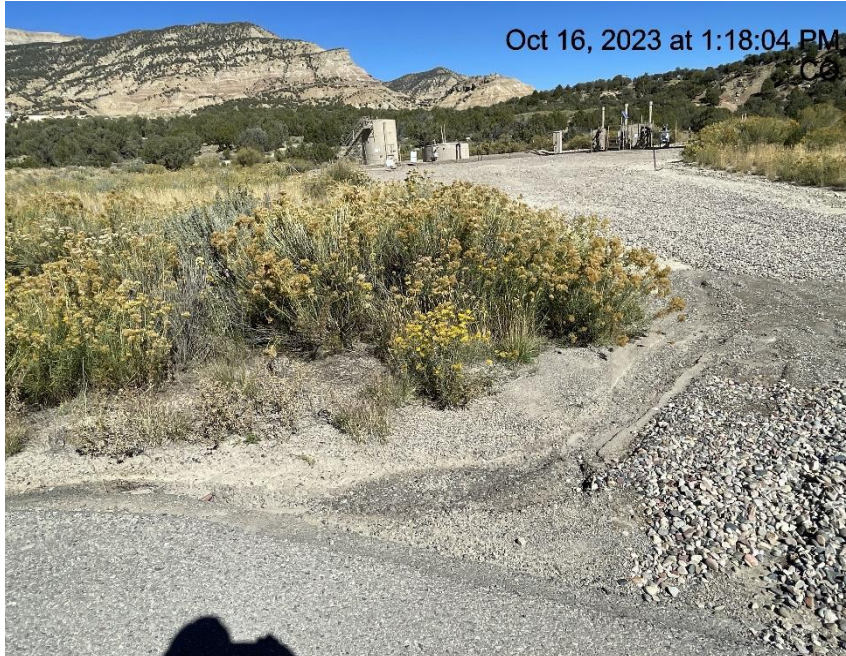
Photo # 2884 From inspection 708901973 conducted on 10/16/2023 Sediment migrating onto gravel track pad/BMP needs maintenance
