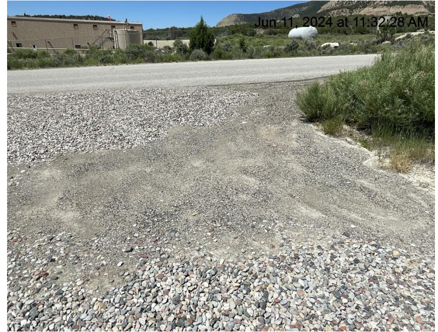
Photo # 442 Sediment migrating onto gravel track pad/BMP needs maintenance
