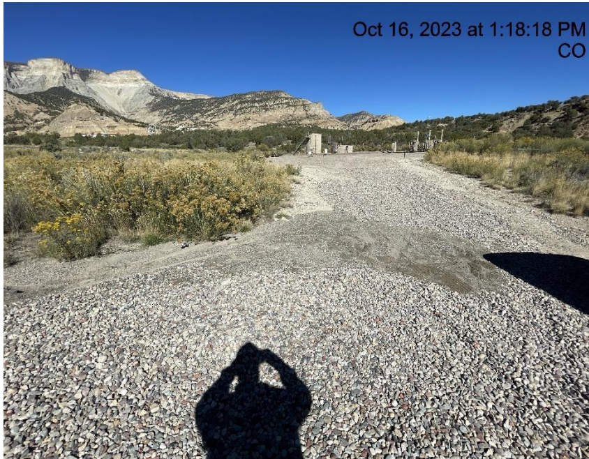
Photo # 2887 From inspection 708901973 conducted on 10/16/2023 Sediment migrating onto gravel track pad/BMP needs maintenance
