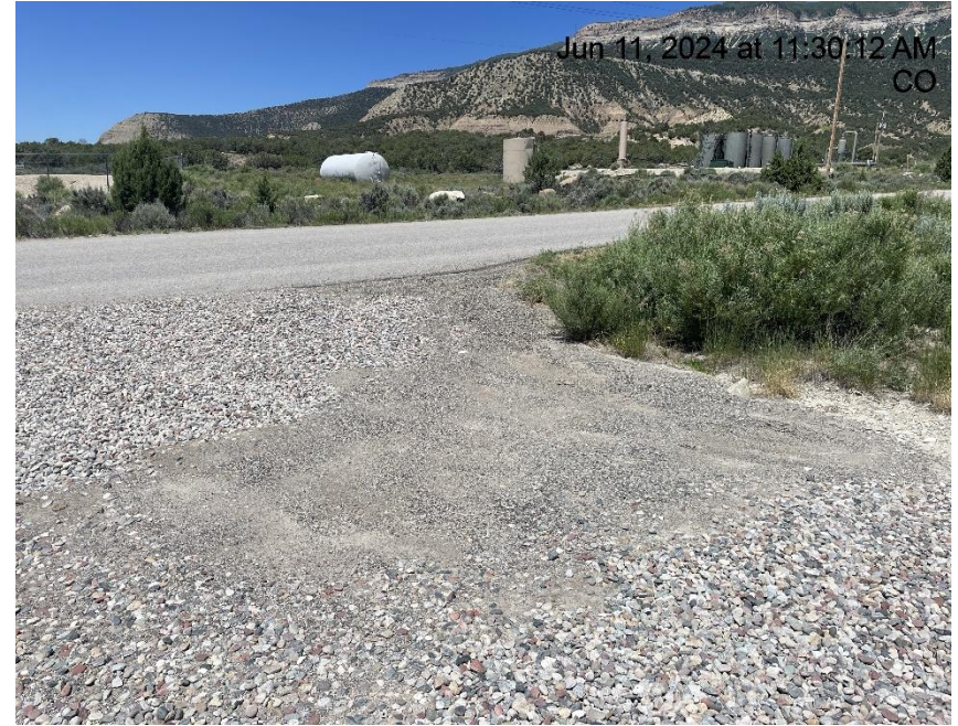
Photo # 439 Sediment migrating onto gravel track pad/BMP needs maintenance
