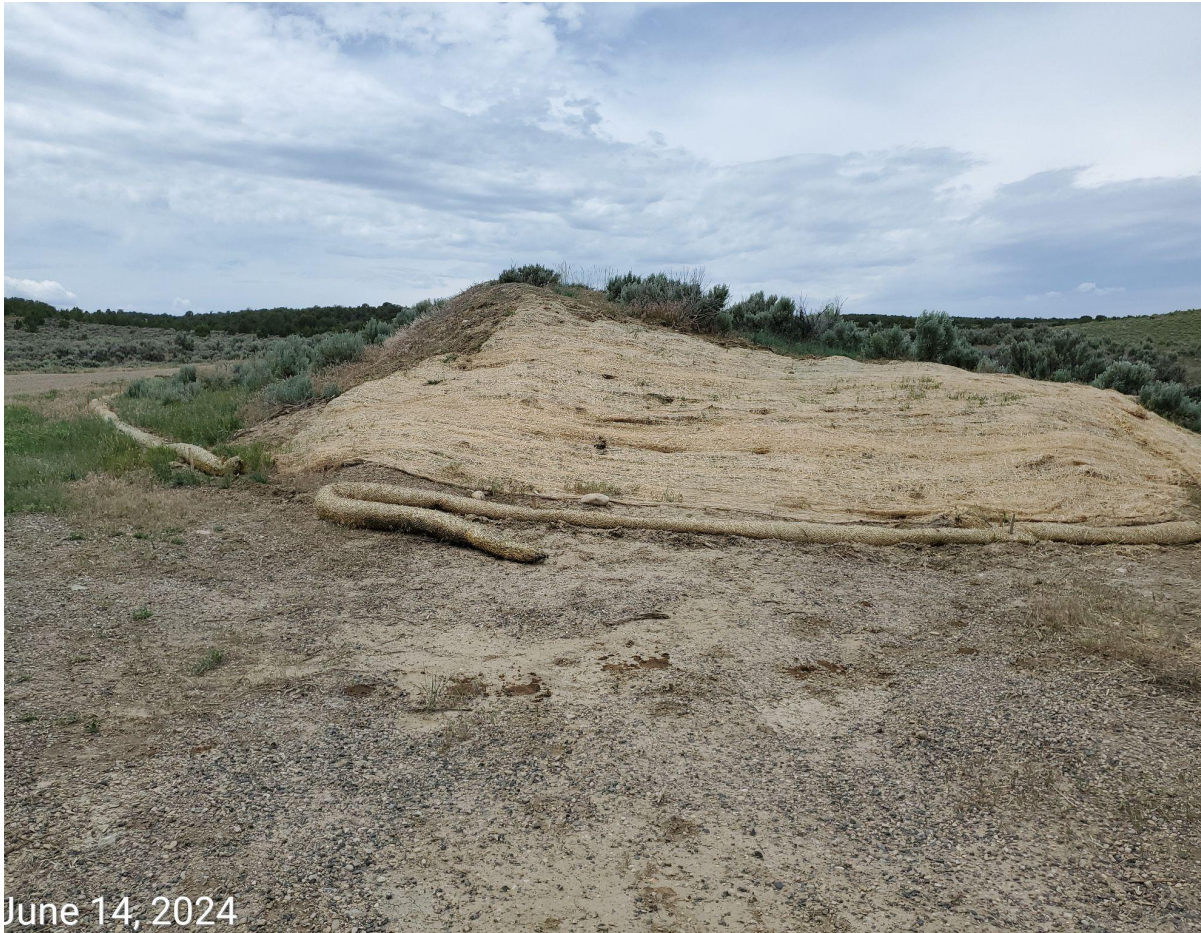
Photo 1: Photo shows soil stockpile on the south end of the Location.
