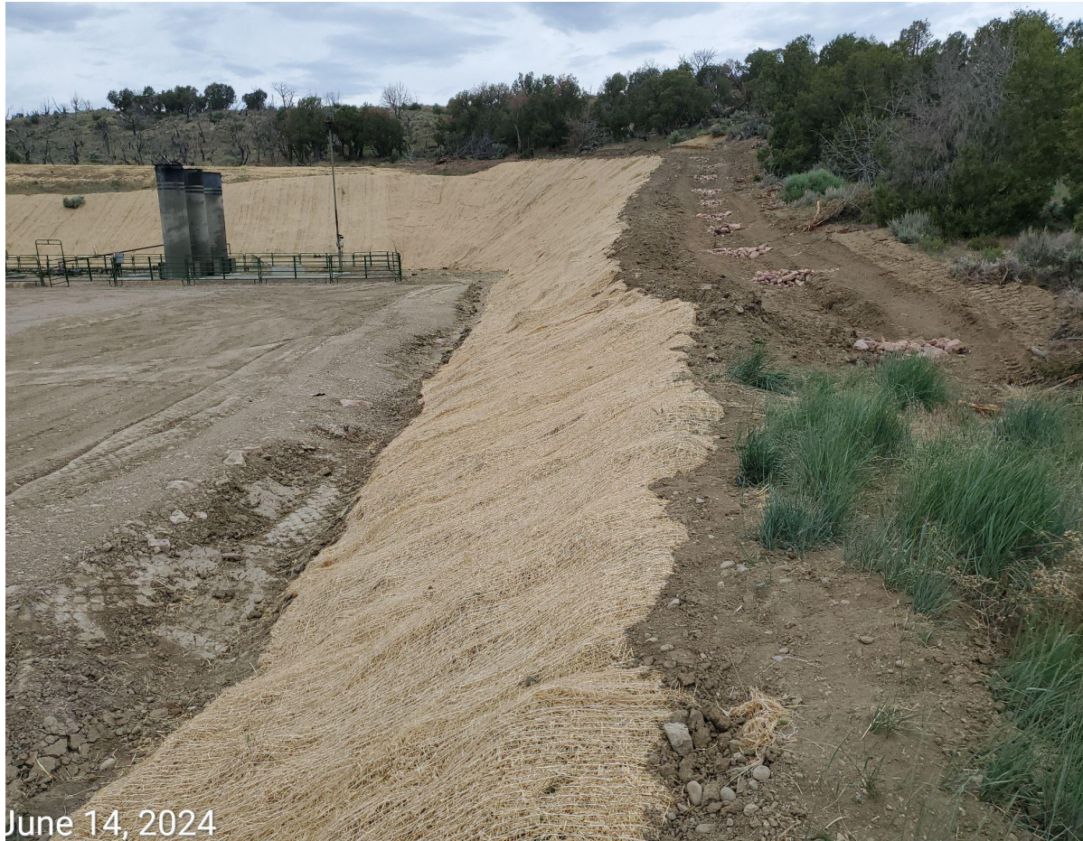
Photo 8: Erosion blankets implemented along cut slopes. Stormwater diversion ditch w/ rock checks implemented.
