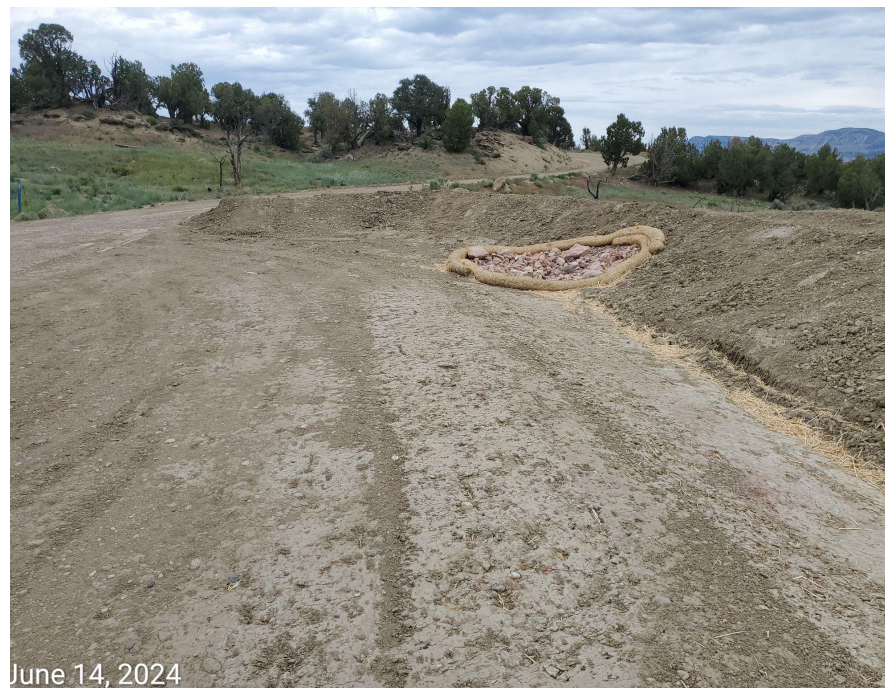
Photo 6: Photos examples showing the slope drains installed on the southeast and northeast ends of the Location.
