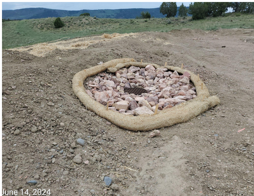
Photo 6: Photos examples showing the slope drains installed on the southeast and northeast ends of the Location.
