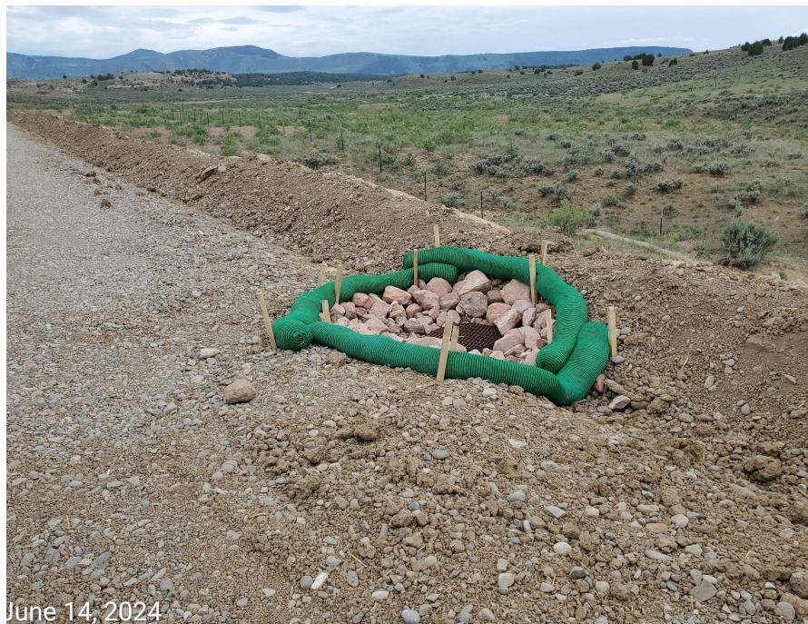
Photo 6: Photos examples showing the slope drains installed on the southwest and northwest ends of the Location.
