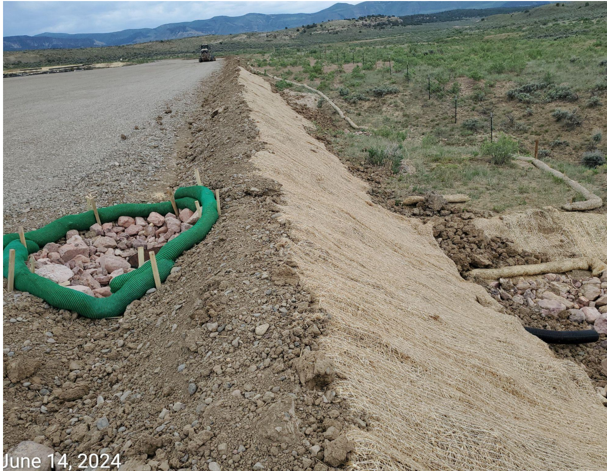
Photo 6: Erosion blankets implemented along portions of the fill slope.
