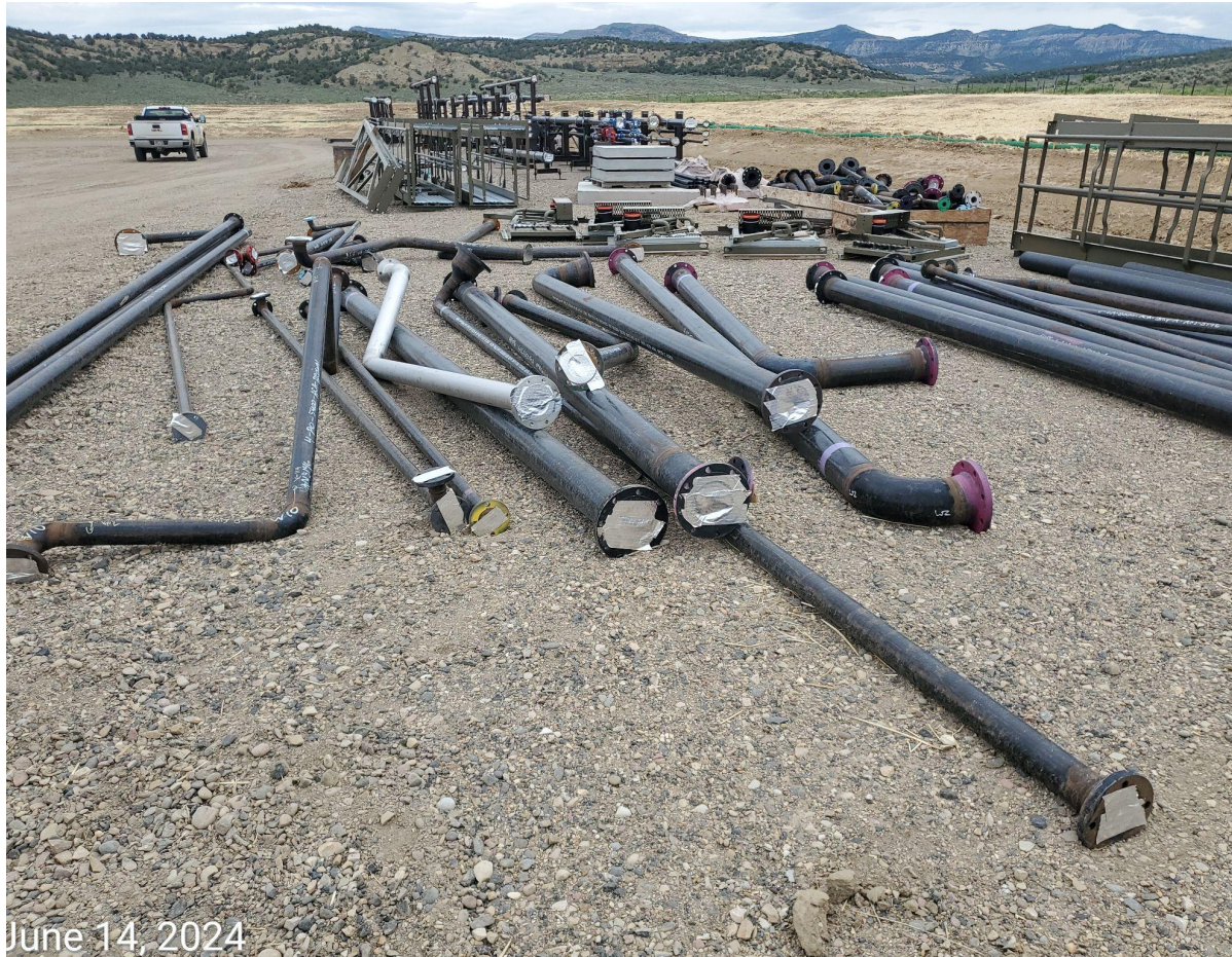
Photo 4: Pipe equipment covered/taped to prevent wildlife access.
