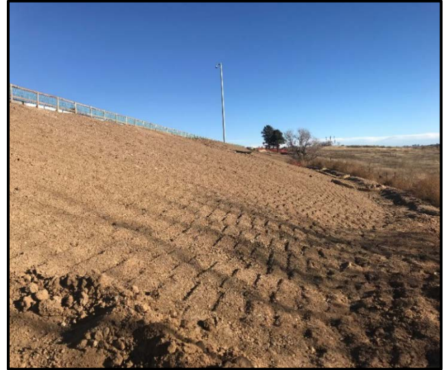
Vertical tracking on disturbed side slope
