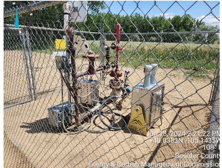
Photo 2 well head and equipment
