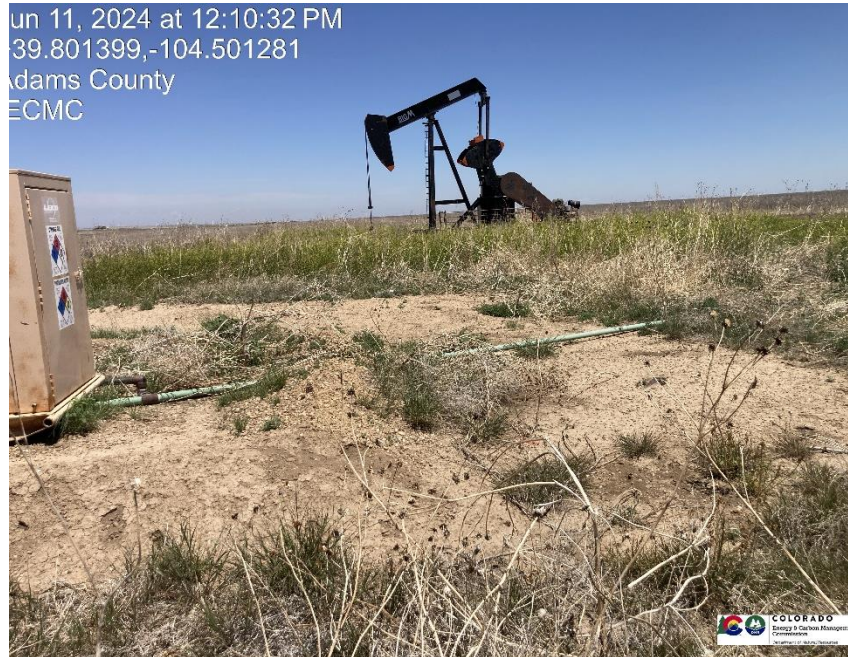
Pic 5 flowline going to separator
