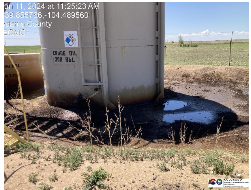
Pic 4 Oil tank, contaminated soil in containment
