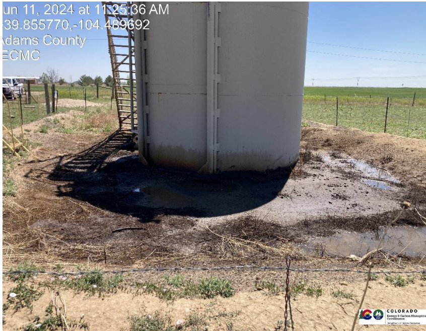
Pic 5 contaminated soil in tank containment
