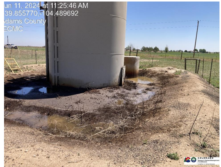
Pic 6 contaminated soil in tank containment
