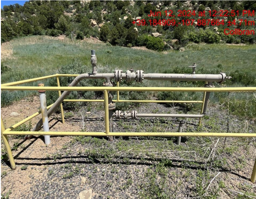
Pig launcher - Photo #02486
