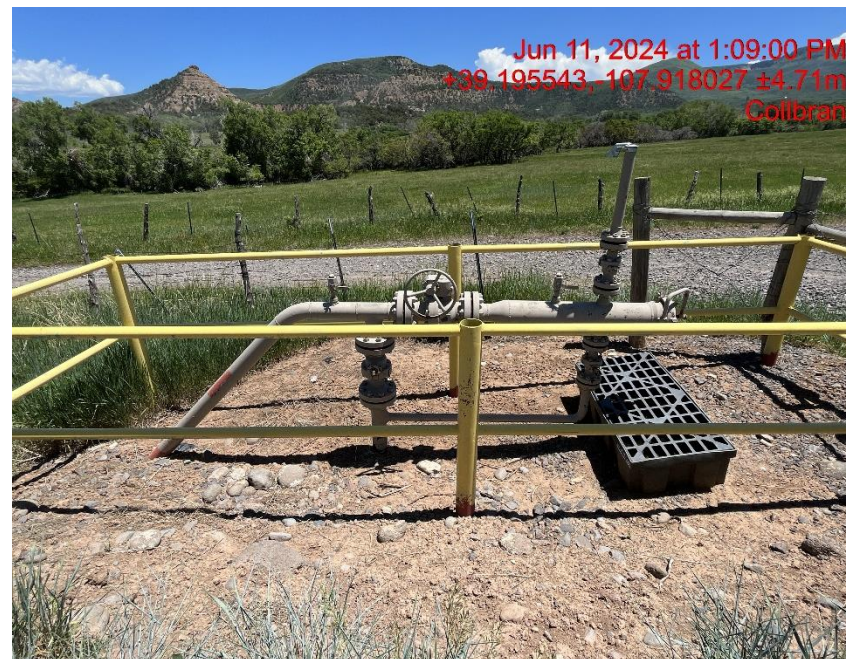
Pig launcher - Photo #02424
