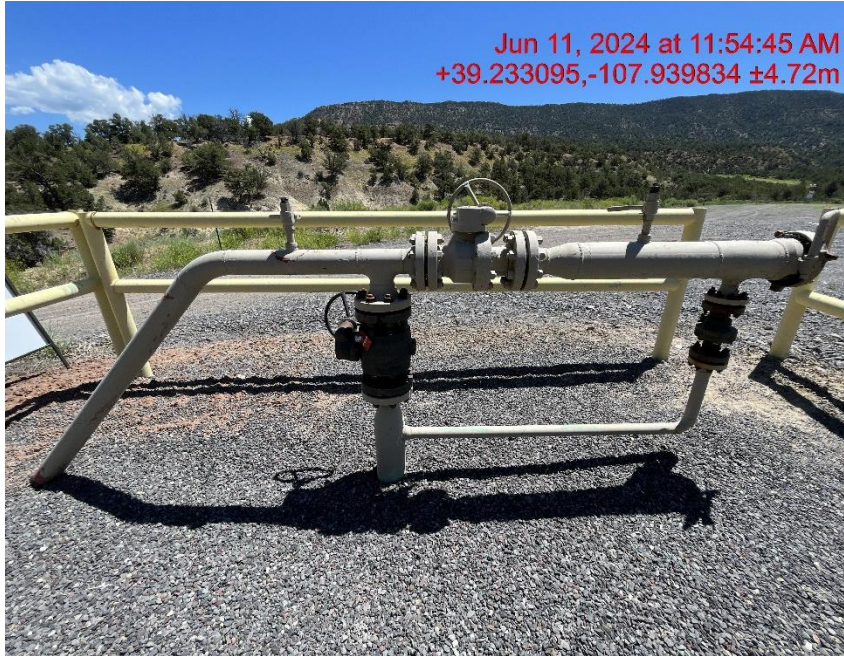
Pig launcher - Photo #02390
