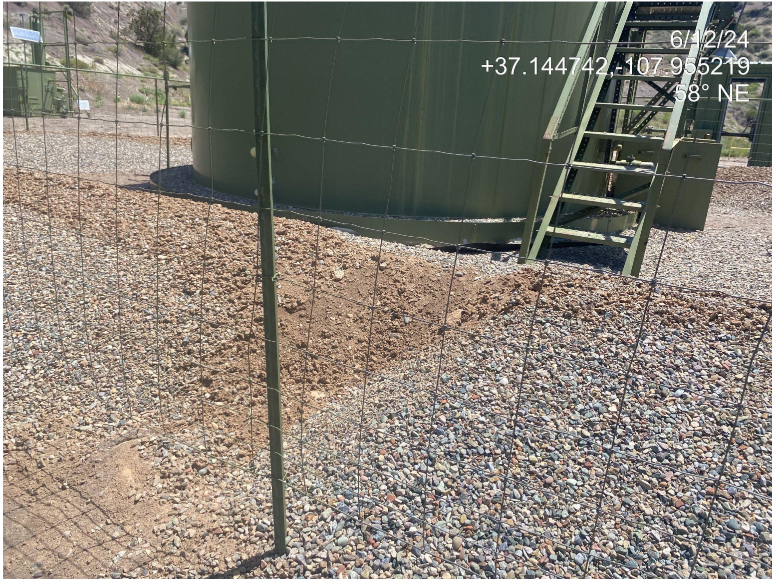
Photo 4. Tank berm remains damaged, maintenance is needed.
