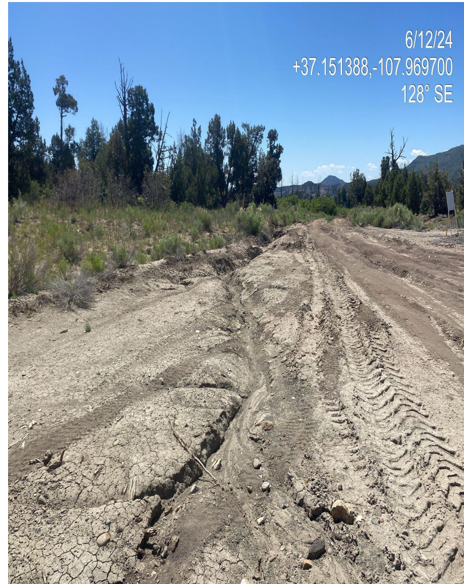
Photo 2. View of erosion forming along at the access point of the disturbance. Additional stabilization/BMPs are needed in this area.
