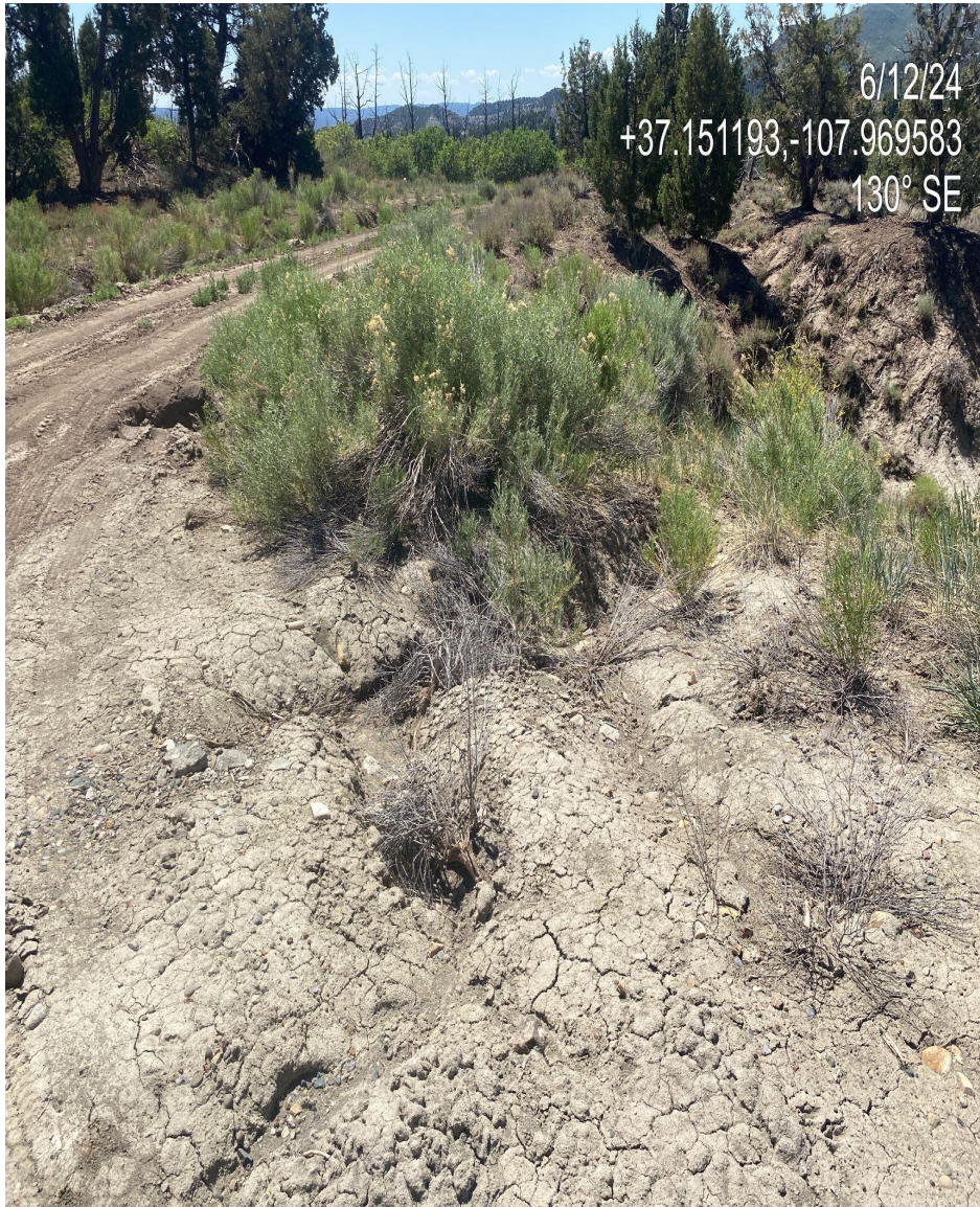
Photo 2. View of erosion forming along at the access point of the disturbance. Additional stabilization/BMPs are needed in this area.
