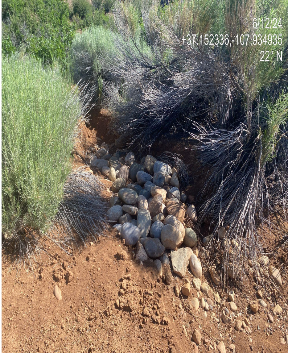
Photo 5. View of round river rock check dam storm water BMP on location on the northern edge of the disturbance. BMP does not appear affective/adequate as gully erosion is persisting down hill.
