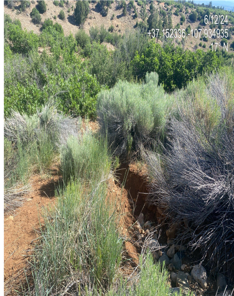
Photo 5. View of round river rock check dam storm water BMP on location on the northern edge of the disturbance. BMP does not appear affective/adequate as gully erosion is persisting down hill.
