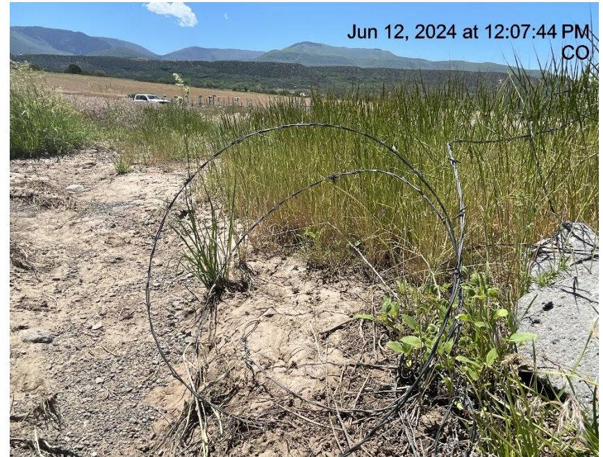
Photo # 557 Barbed wire fence needs maintenance/wildlife hazard
