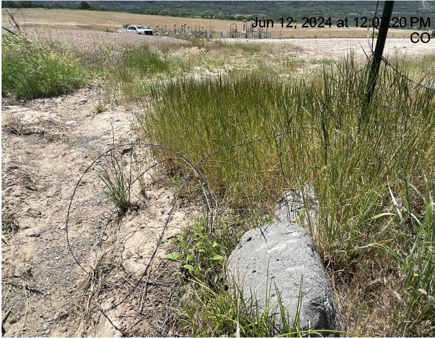
Photo # 554 Barbed wire fence needs maintenance/wildlife hazard
