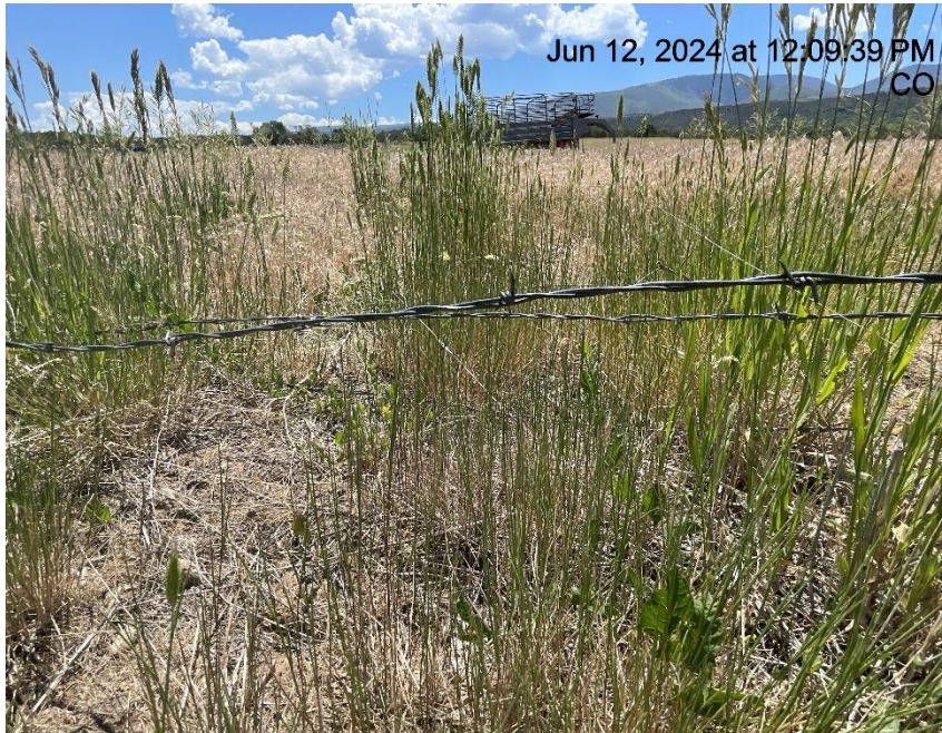
Photo # 562 Barbed wire fence needs maintenance/wildlife hazard
