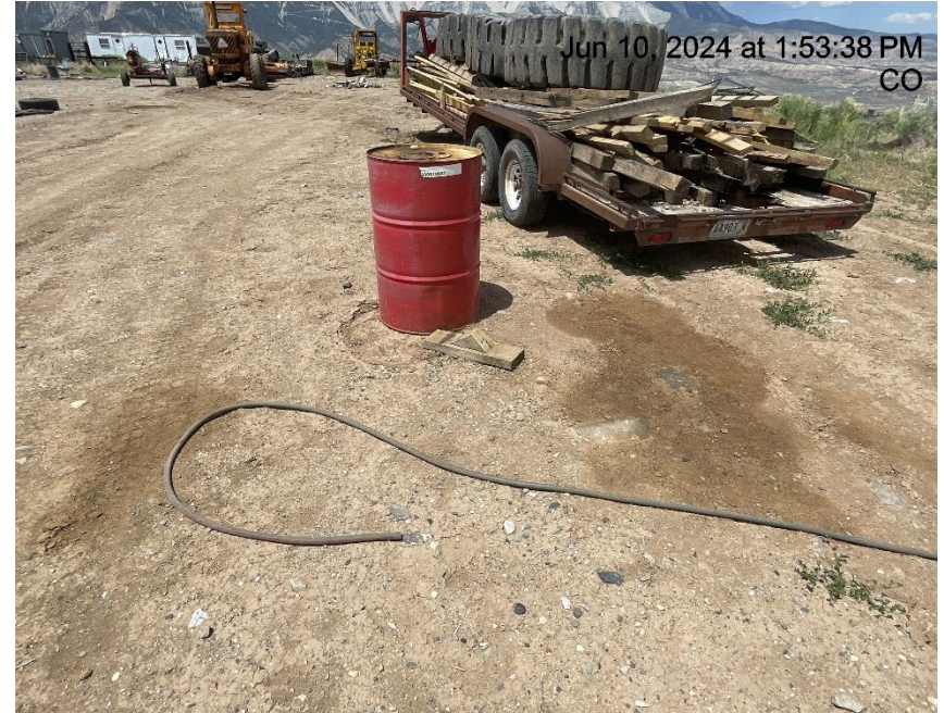
Photo # 307 Chemical drum with no BMP's
