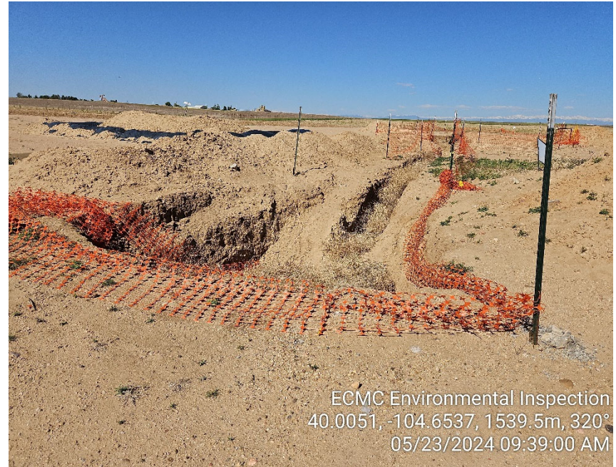
Photo 20 – Open excavation; downed fencing.
