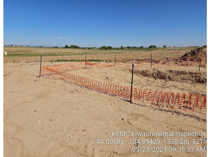
Photo 4 – Open excavation; sagging fencing.
