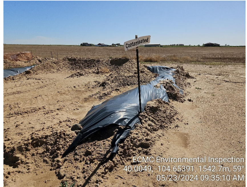
Photo 16 – Contaminated soil stockpile.
