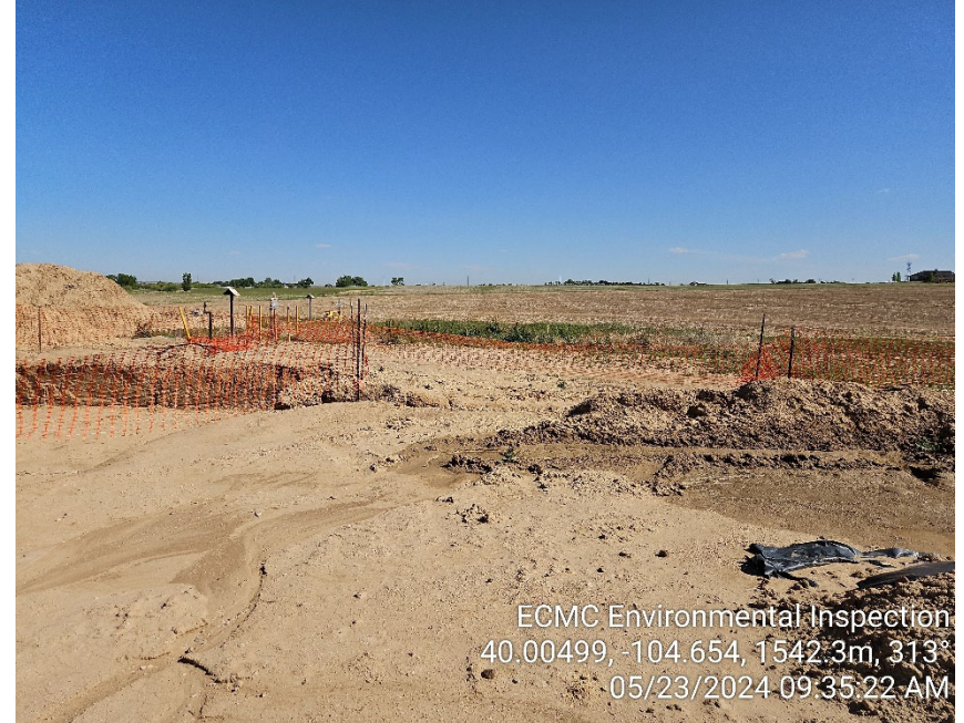
Photo 2 – Open excavation; downed fencing.
