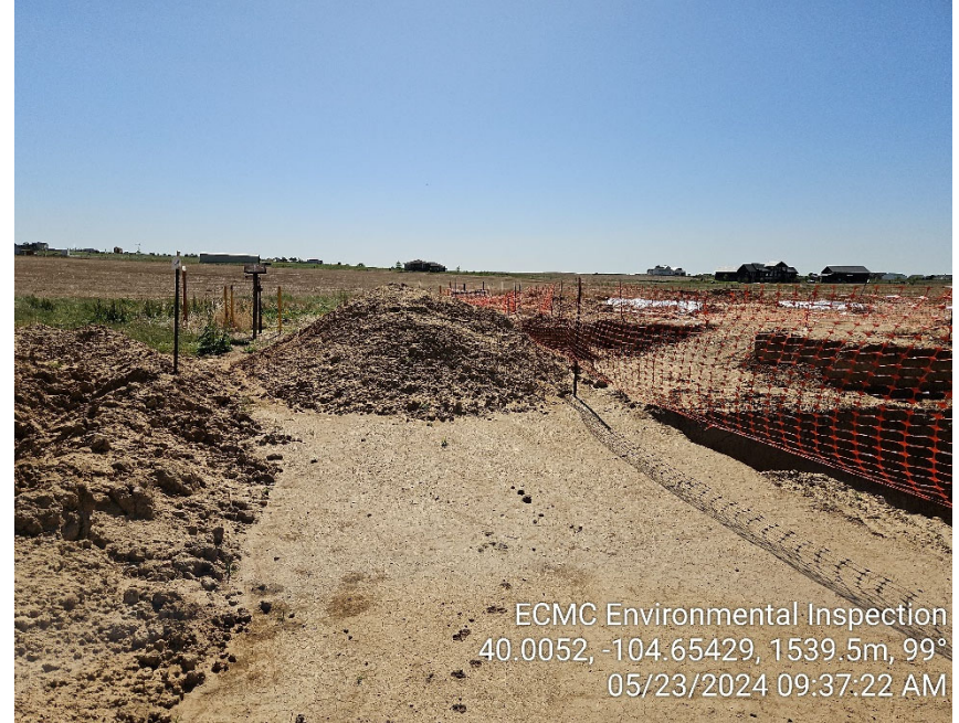
Photo 10 - Small soil stockpile; unmarked with no BMPs
