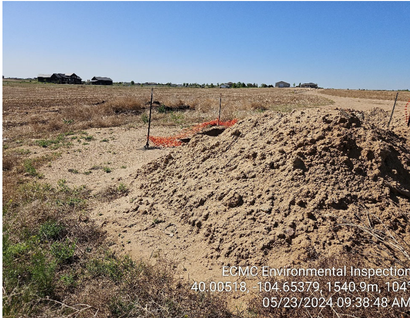
Photo 19 – Small unmarked soil stockpile with no BMPs. Downed fencing.
