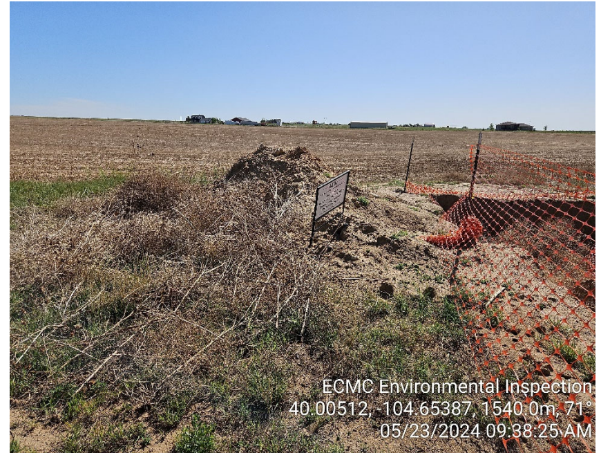
Photo 12 - Small soil stockpile; unmarked with no BMPs
