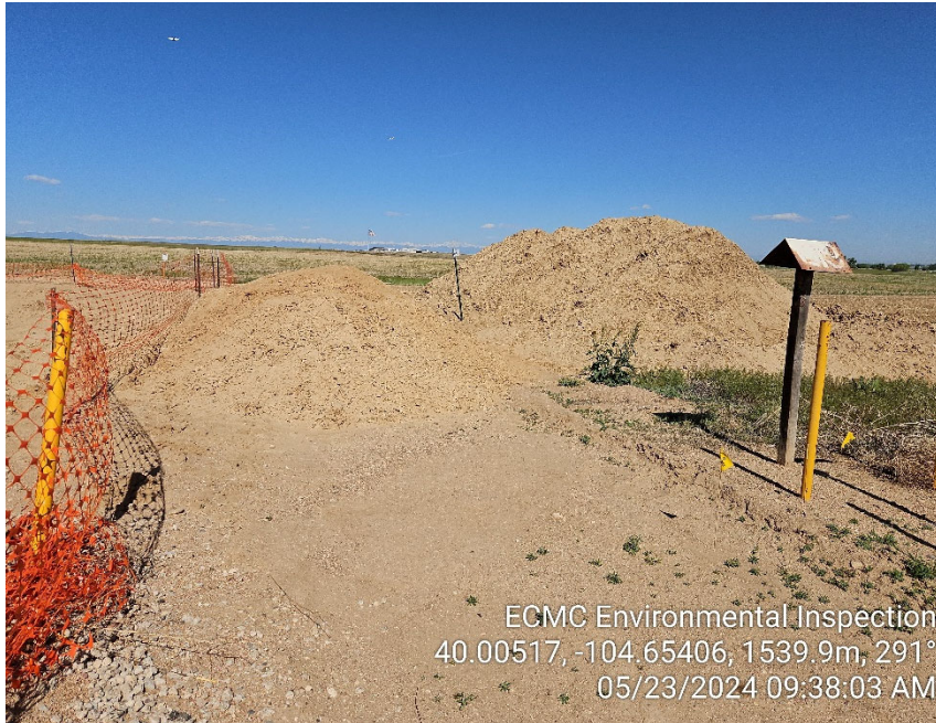
Photo 11 - Small soil stockpile; unmarked with no BMPs (foreground). Large clean soil stockpile (background).
