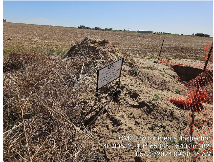
Photo 14 - Small soil stockpile; unmarked with no BMPs
