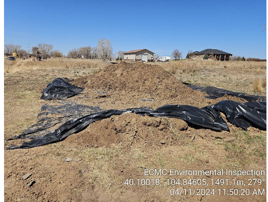
Photo 4 - Soil stockpile on liner and bermed.
