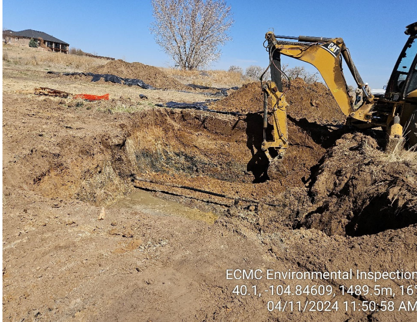
Photo 5 – Groundwater observed in open excavation. Impacts remained visible in-situ.
