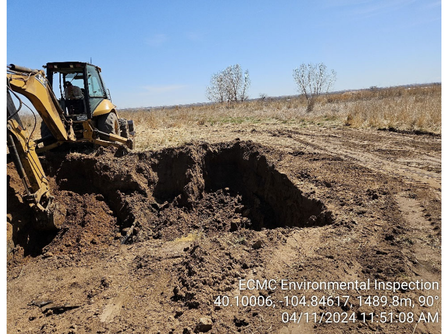
Photo 6 - Groundwater observed in open excavation. Impacts remained visible in-situ.
