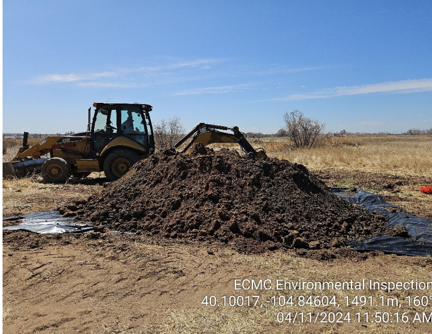
Photo 3 – Soil excavated from spill area temporarily stored on tarp. Contaminated soil beginning to overtop onto clean soil
