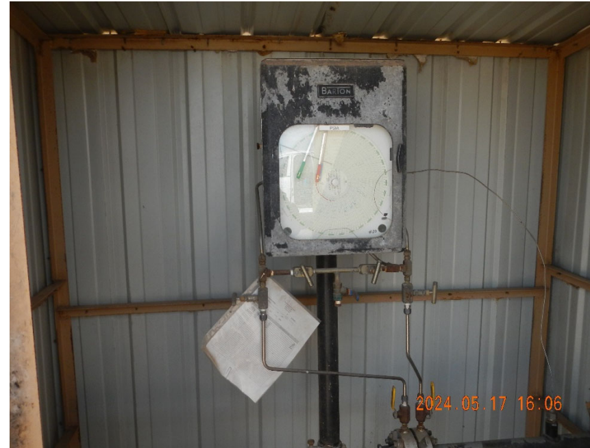
8. Gas meter inside meter shed.
