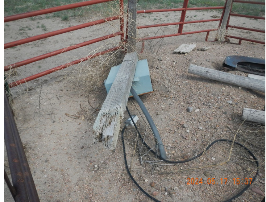
4. Power and control panel laying on ground.
