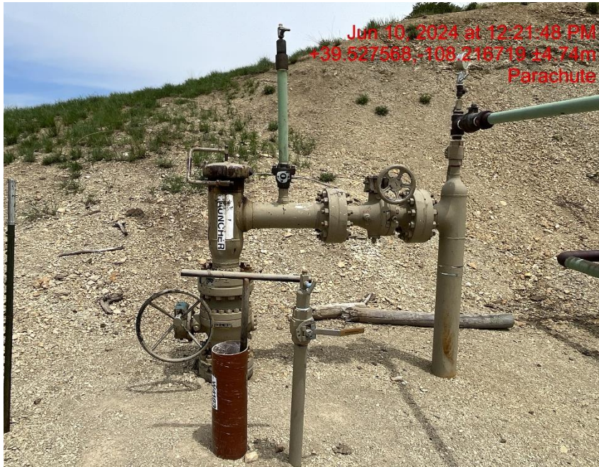
Pig launcher - Photo #02291
