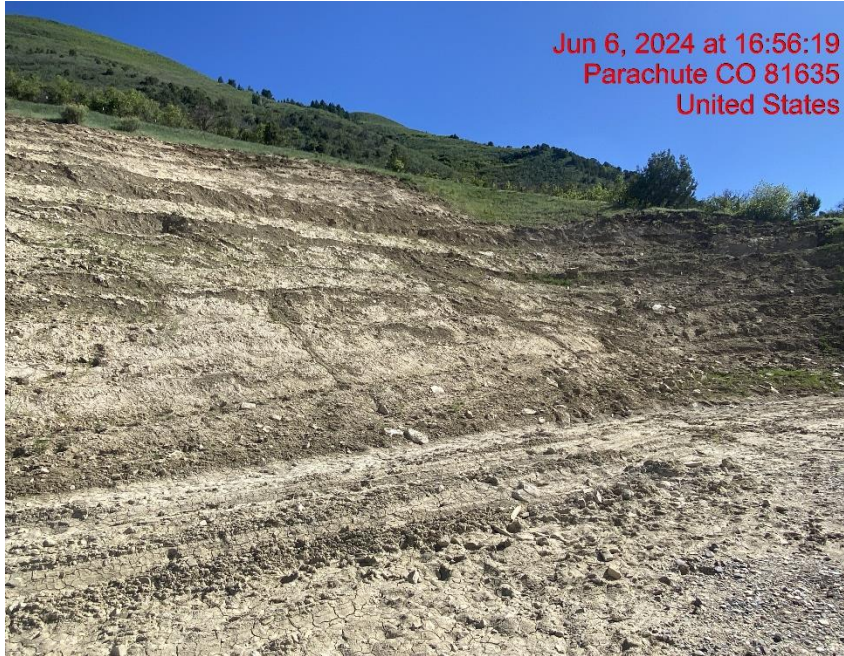
Insufficient Erosion Control onto Location – Photo #01648
