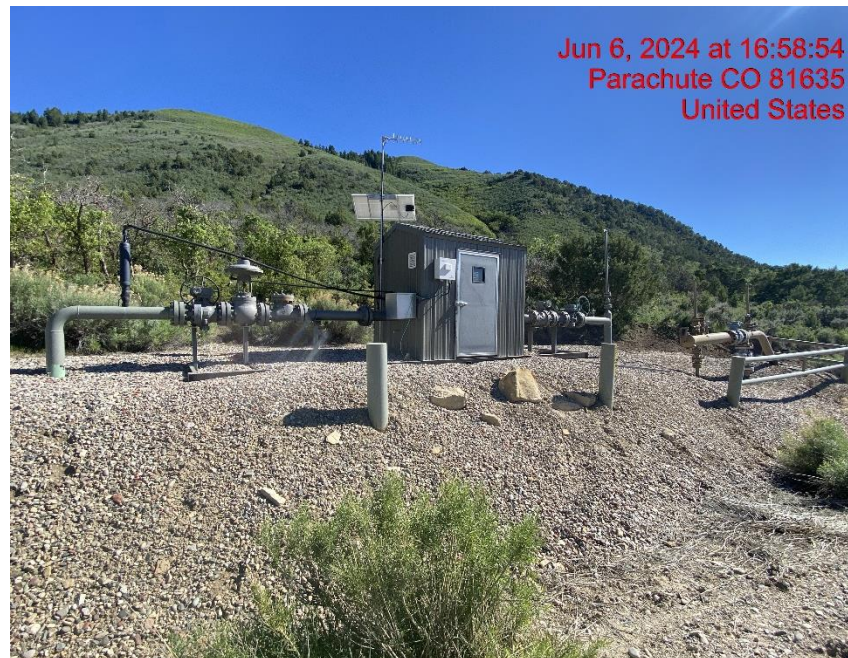
Gas Meter/Pig Station – Photo #01653
