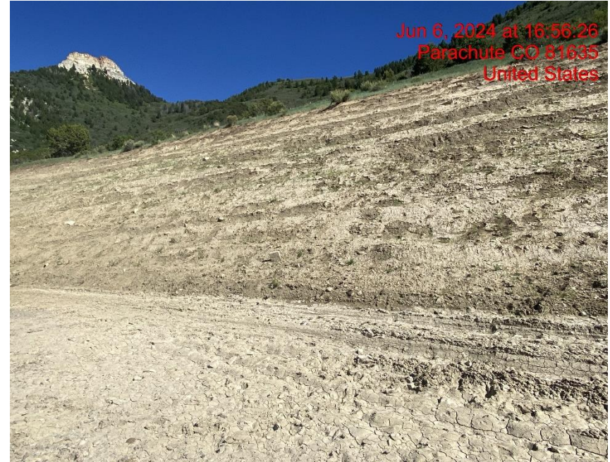
Insufficient Erosion Control onto Location – Photo #01649
