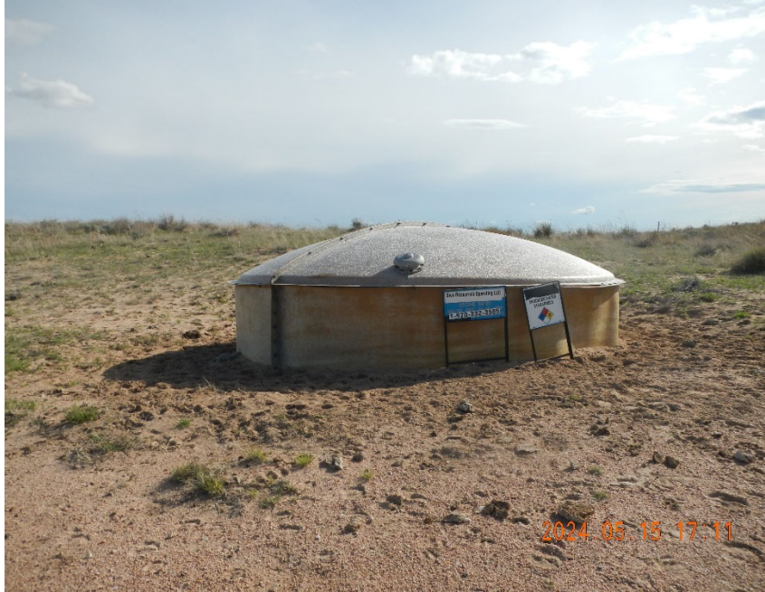
3. View of produced water tank.
