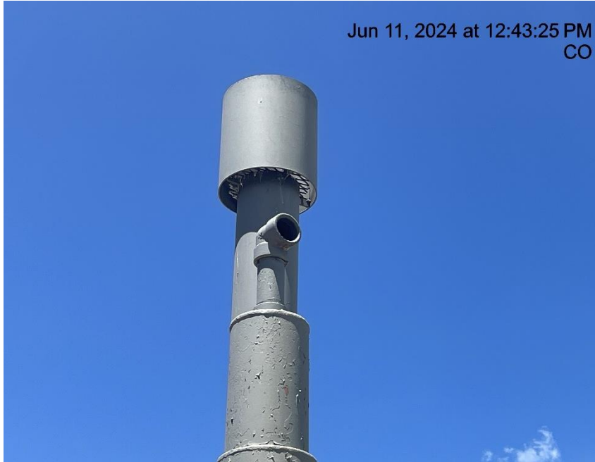
Photo # 506 Open ended piping on separator/wildlife hazard/available for entry by wildlife
