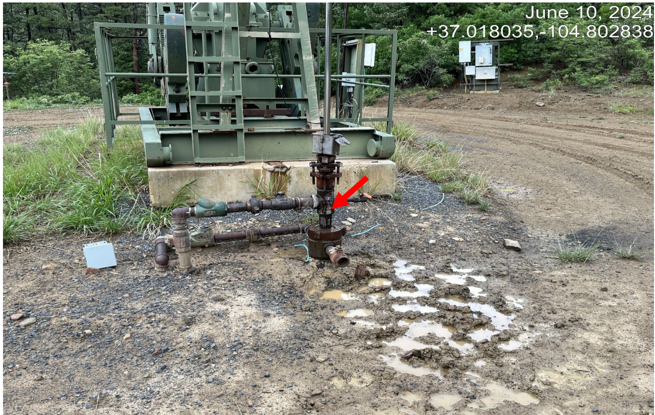
Photo 4. The wellhead has a dripping leak.
