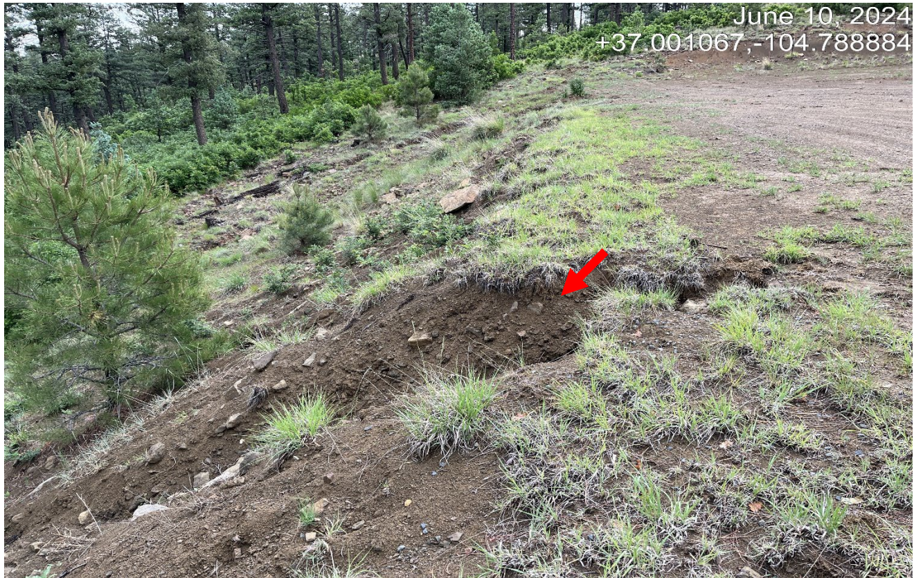
Photo 3. There is an erosion channel at the northwest side of the location that needs to be repaired. Arrow points to 4.5 ft. shovel.
