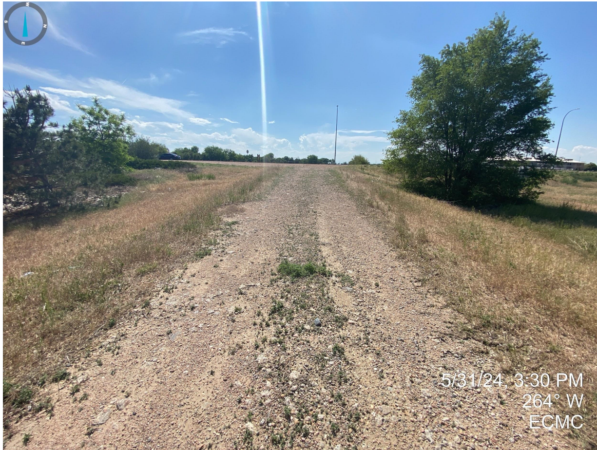
Photo 1. Access road does not appear to have been reclaimed with the presence of road base material.
