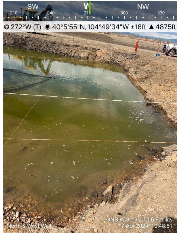
North and West side wall of excavation extent
