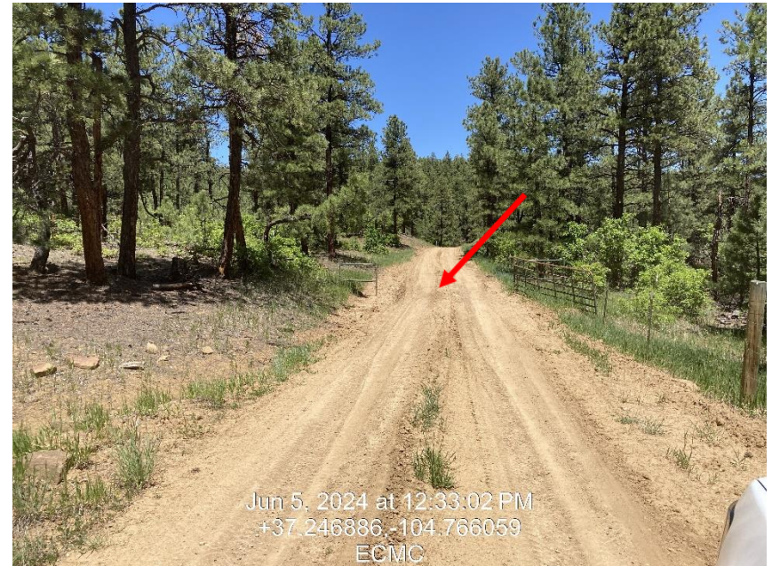
Photo 6 – Access road, vehicle rutting
