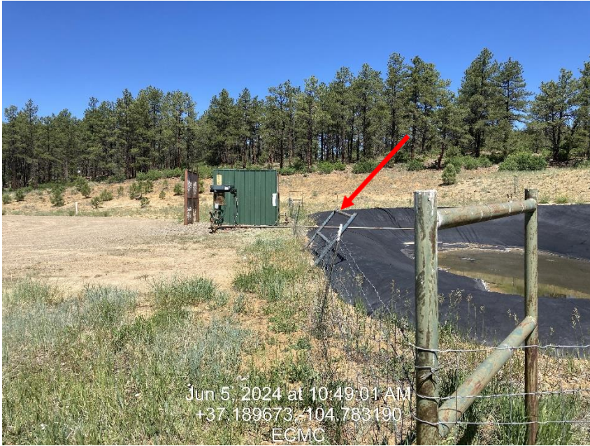
Photo 5 – H-brace on truck load out leaning
