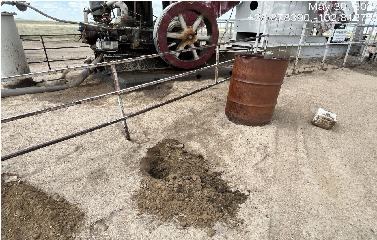
Photo 7. It appears there was sand spread on top of the spill which was not cleaned up per the rules.
