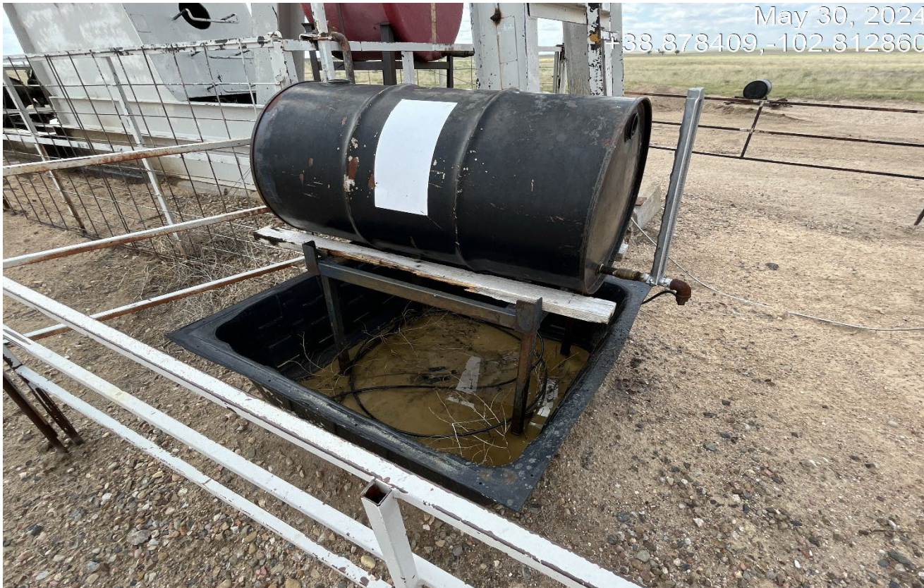
Photo 9. There is oily fluid in the secondary containment and no wildlife protection/netting is installed. The labeling on the barrel is faded and needs to be updated.
