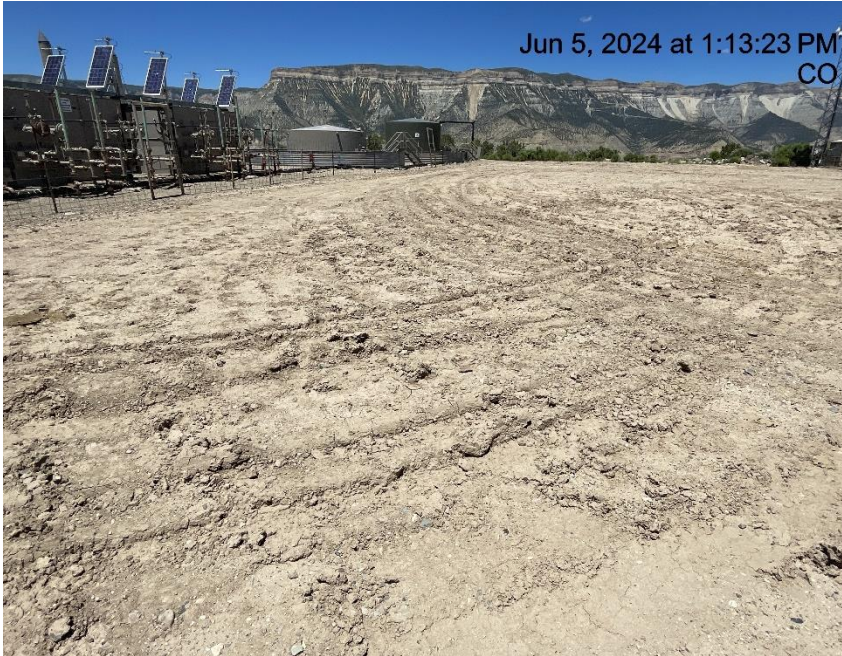
Photo # 9696 Lack of stabilization/compaction
