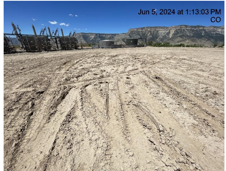
Photo # 9693 Lack of stabilization/compaction
