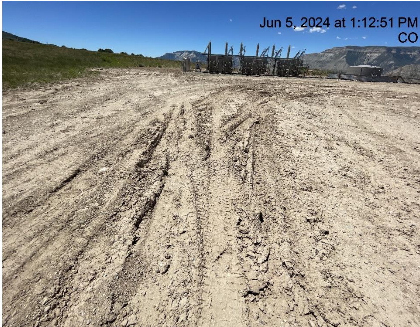
Photo # 9692 Lack of stabilization/compaction
