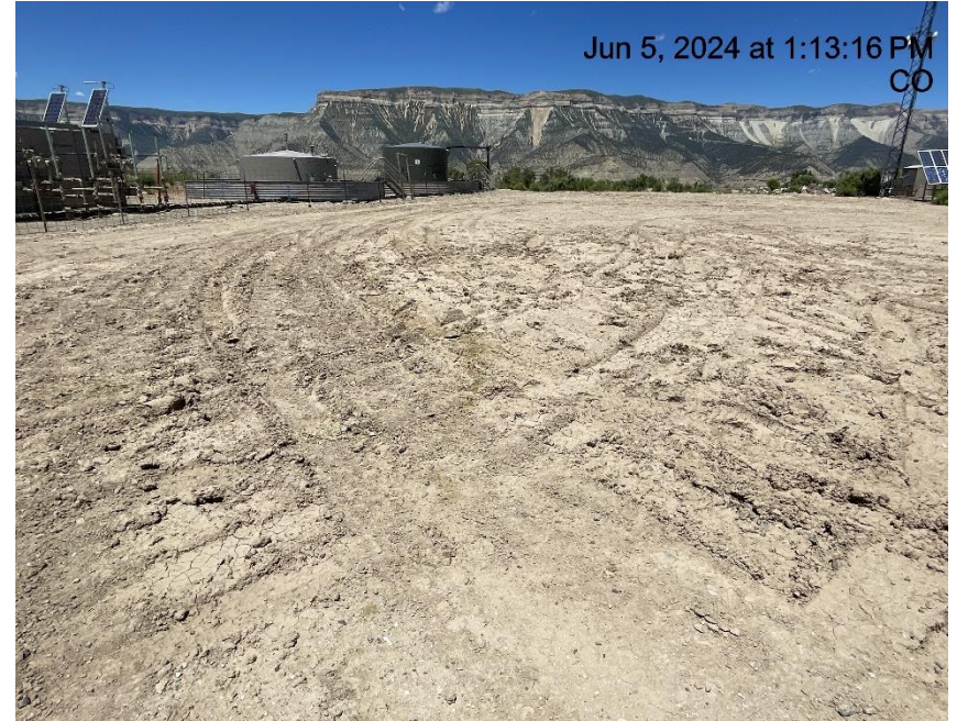
Photo # 9695 Lack of stabilization/compaction
