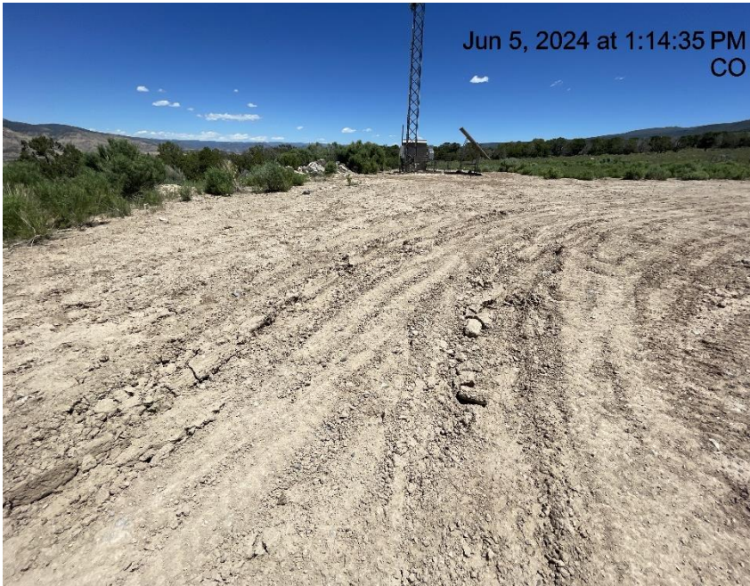
Photo # 9698 Lack of stabilization/compaction
